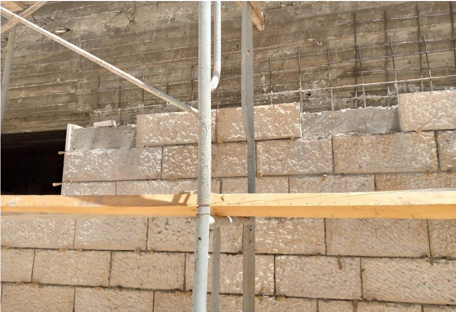
Removing defected stones
