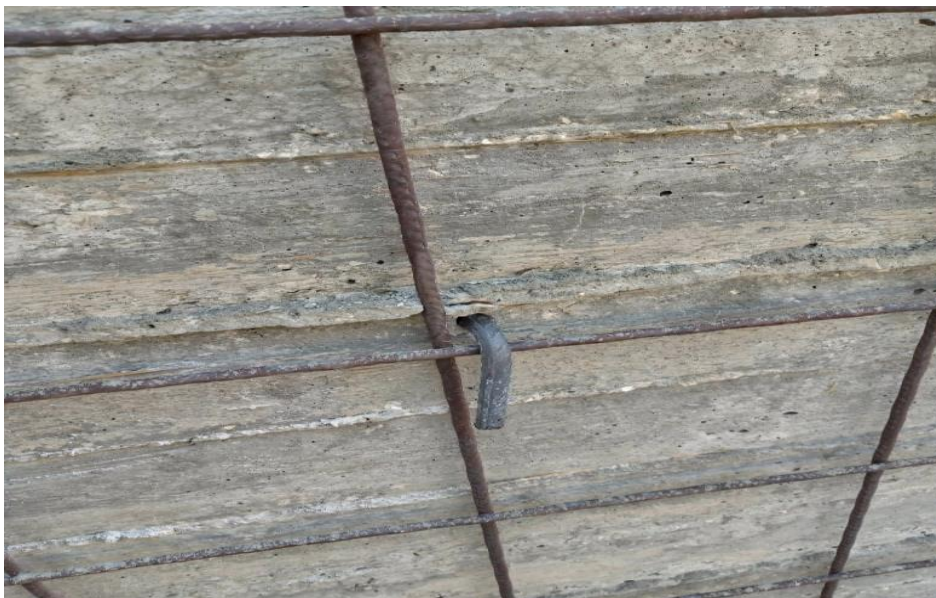
Rectifying the fixation of stones
