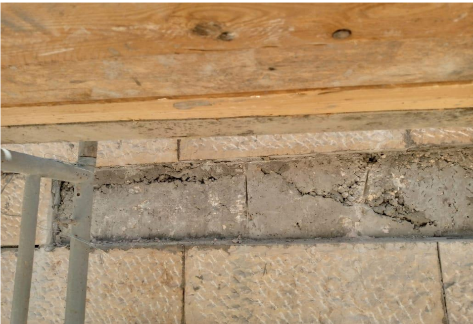
Removing defected stones
