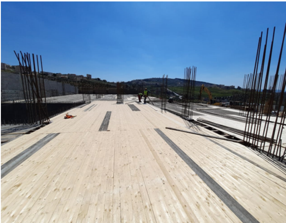
Formwork for ground floor slab part A-D/1-10- (28/03/2021)
