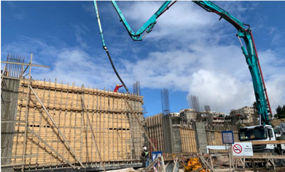
Concrete casting for the main building walls- (04/03/2021)
