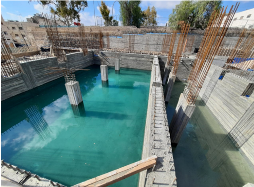
Penetration test for water tank- (03/03/2021)
