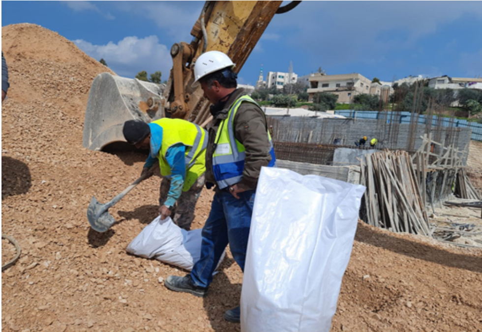
Taking Base course samples by laboratories and quality control department in MPWH- (02/03/2021)
