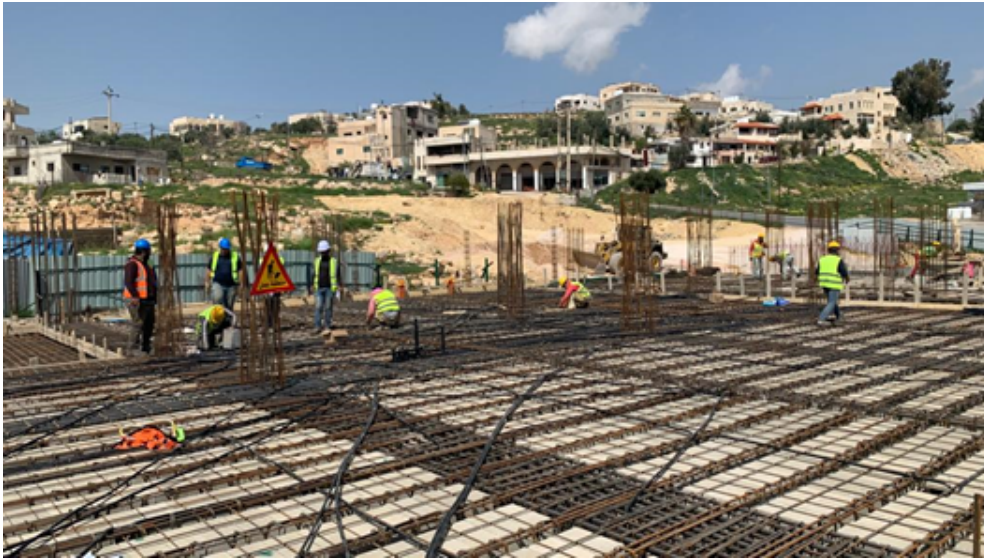
Preparation for main building slab casting- (16/03/2021)
