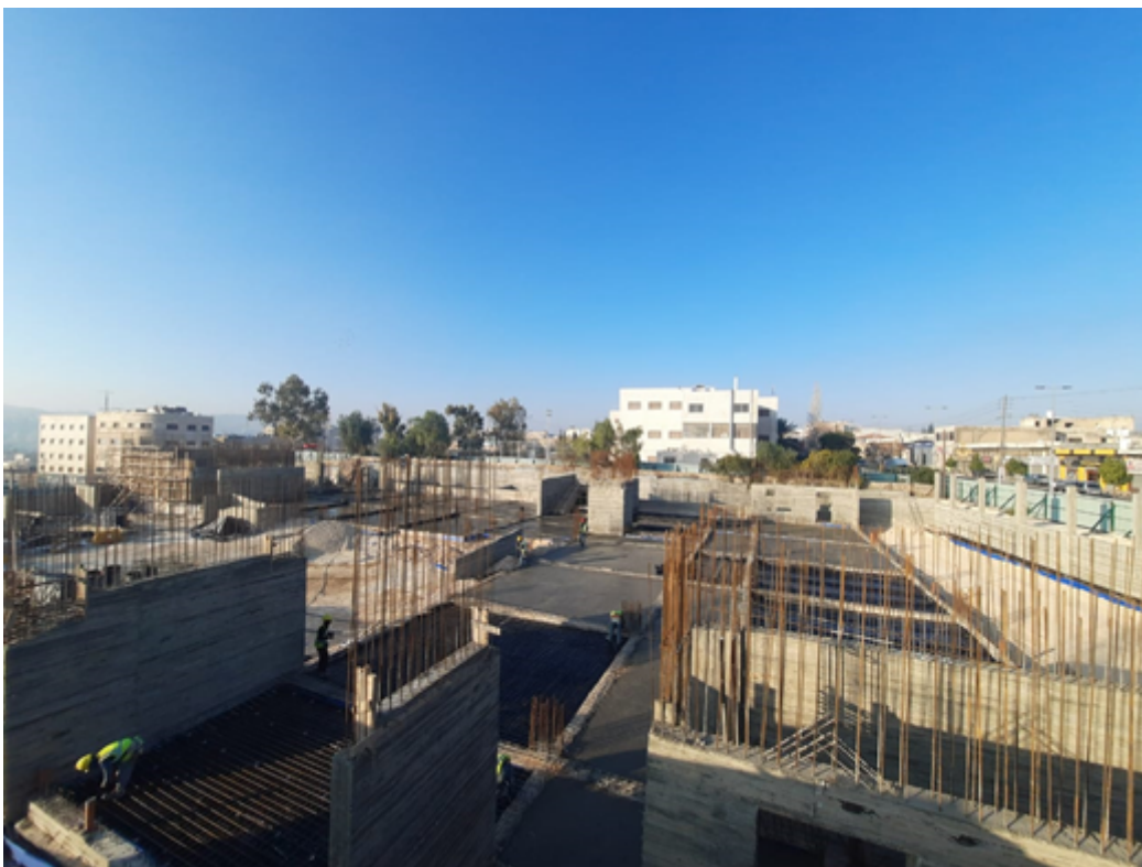
General view of ground floor slab on grade- (28/03/2021)
