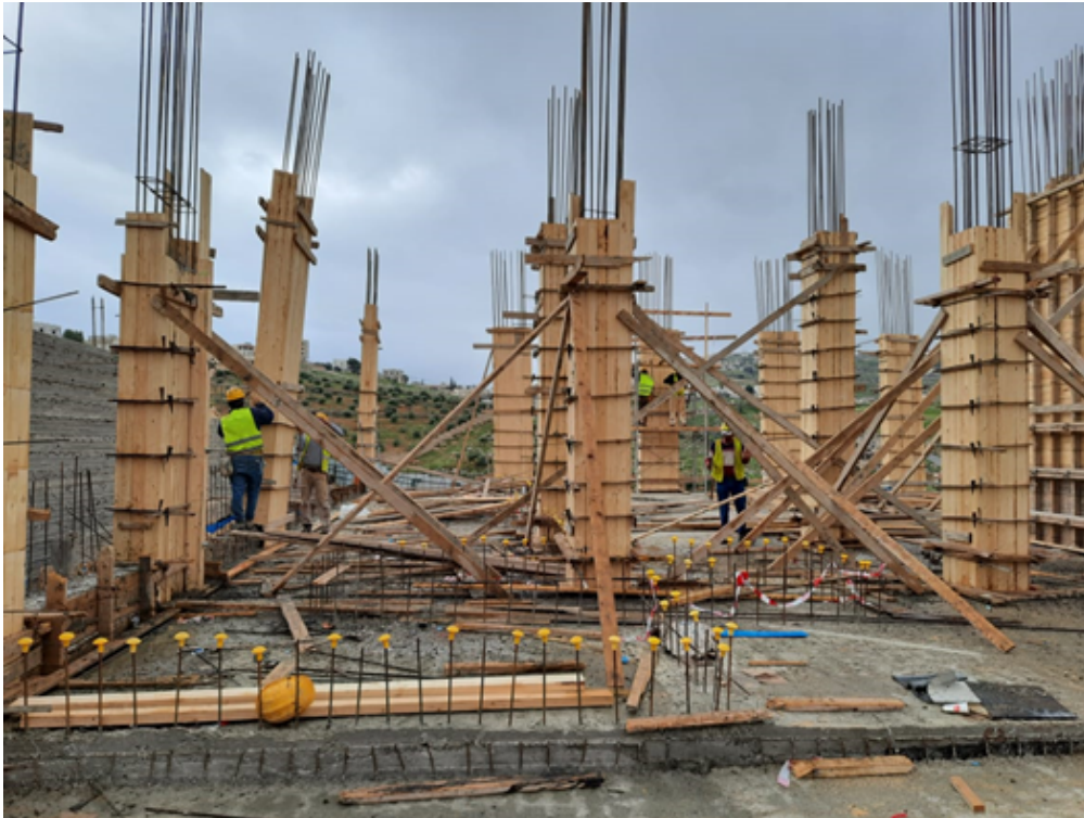
Formwork for ground floor columns- (15/03/2021)
