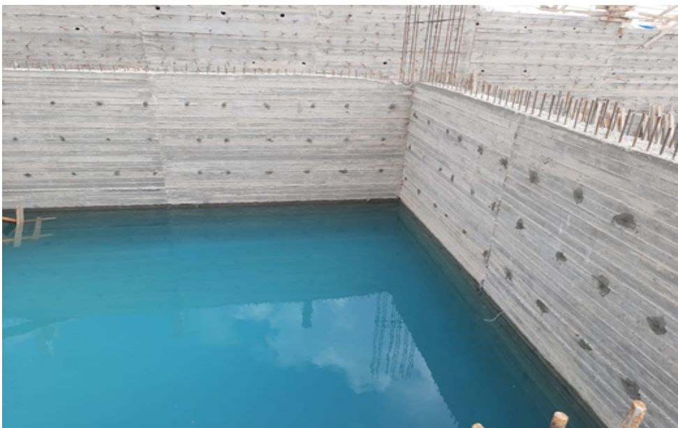
Penetration test for water tank before any treatment- (08/03/2021)
