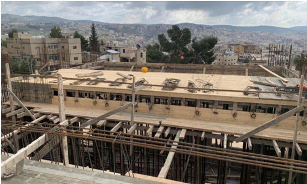
Formwork for theater roof slab- (08/03/2021)
