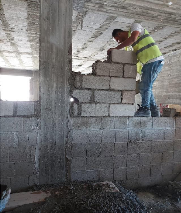
removal of un-complied blockwork
