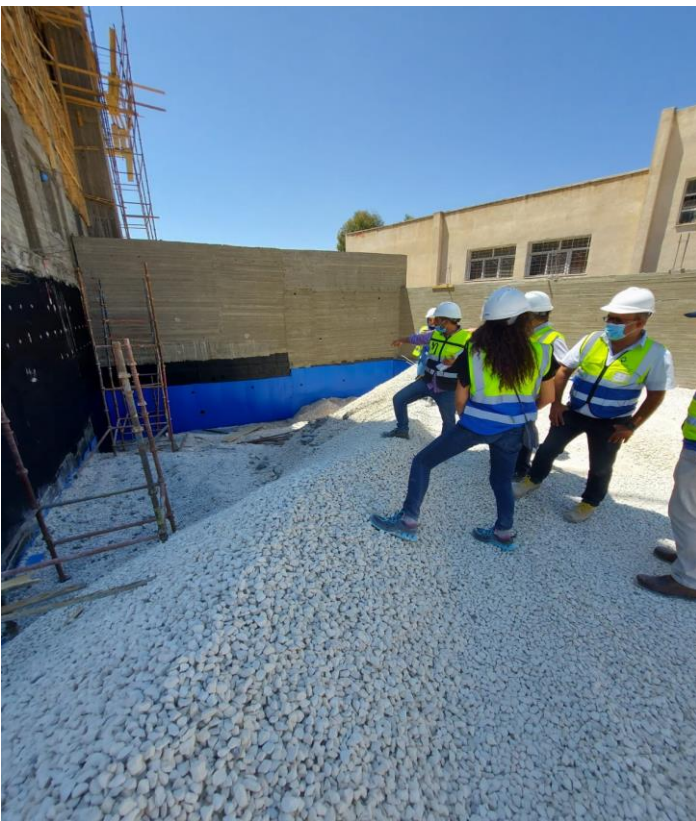
Starting remedy work in the presence of Engineer representatives
