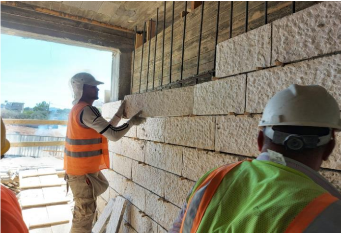
removal of un-complied Stone
