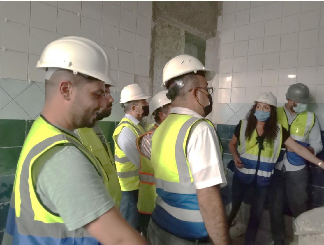
Inspecting Tiling work at the wet area/ground floor
