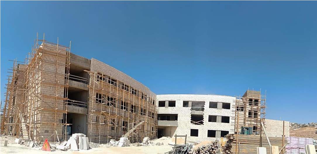
General view of the completed second floor casting (the last slab)
