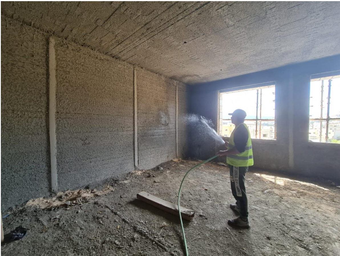
Curing of plastering work
