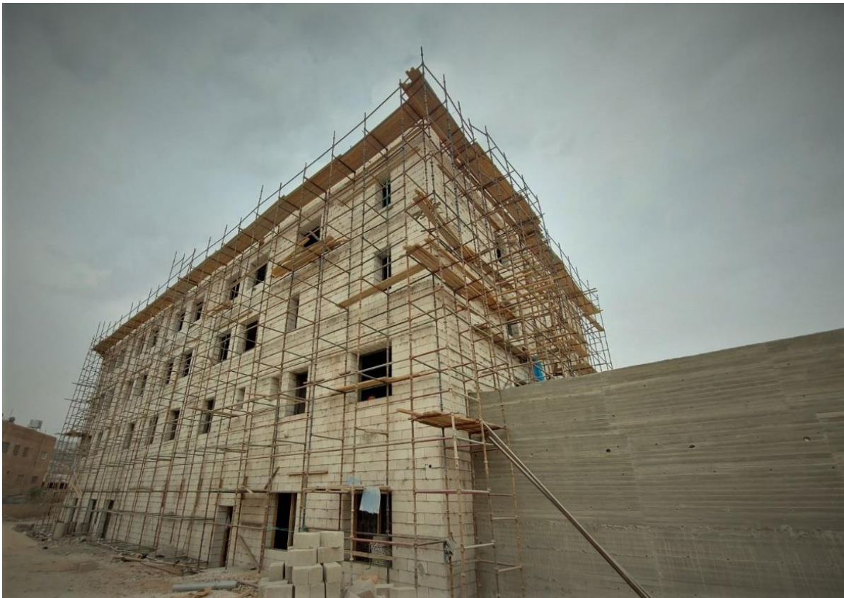
The Supervision team observed the stone building for facades in general
