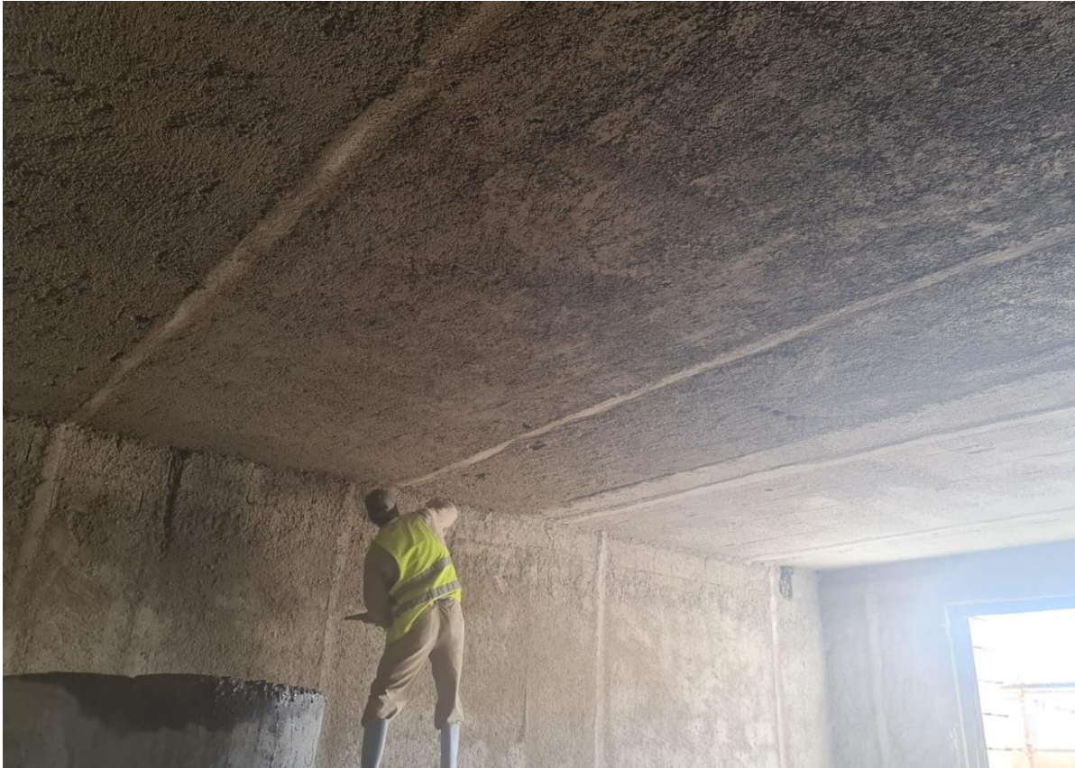
inspecting the process of executing second layer of plaster
