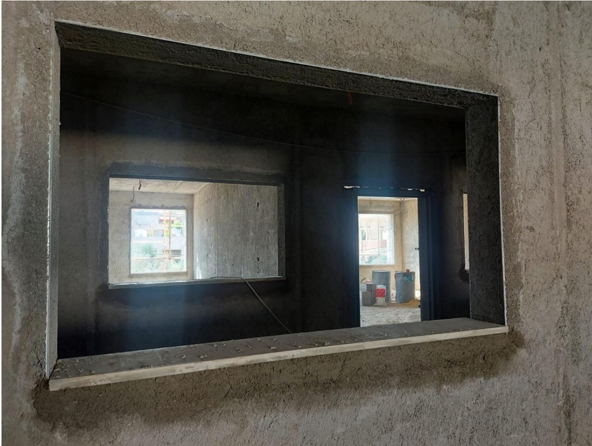
Window Sills installation
