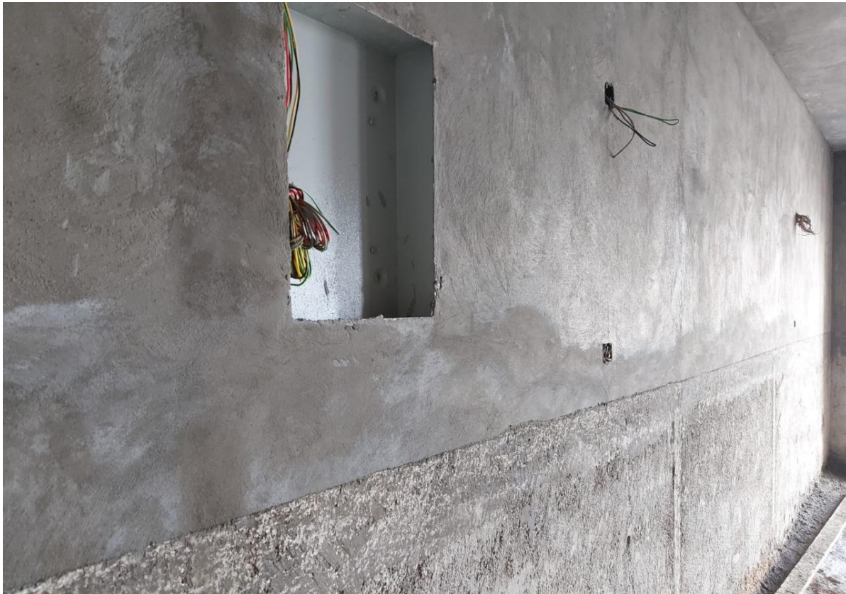
Inspecting the last layer of plastering
