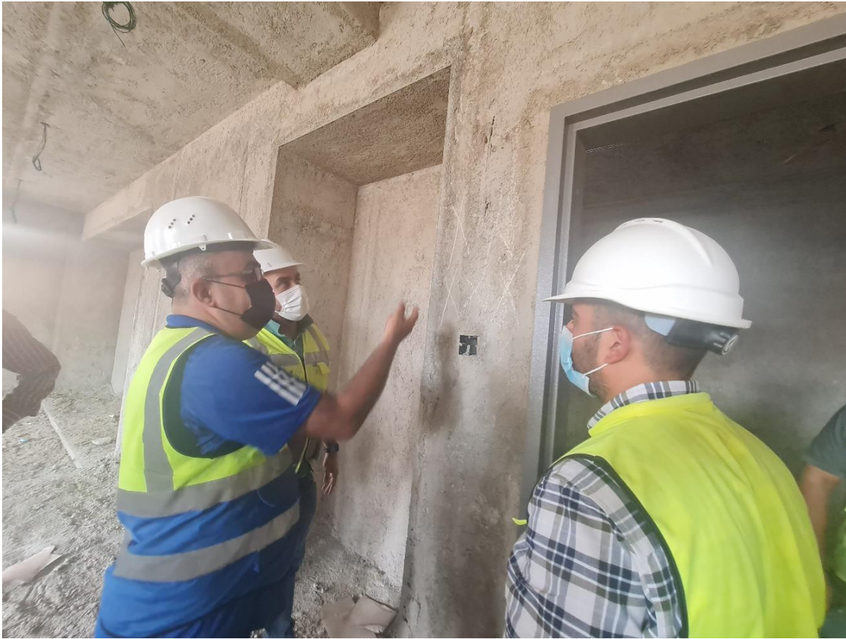
general check on the installed door frames
