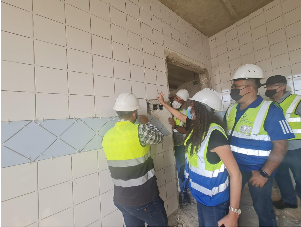
Electrical sockets location was discussed in relation with wall tiles
