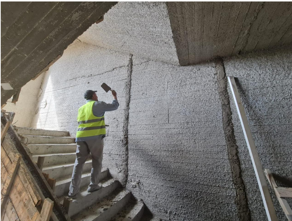
Applying plastering guidelines
