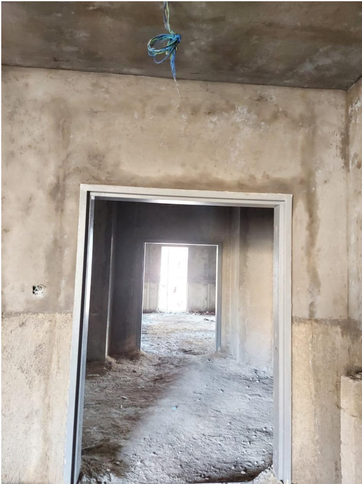
Frames installation for Wooden doors
