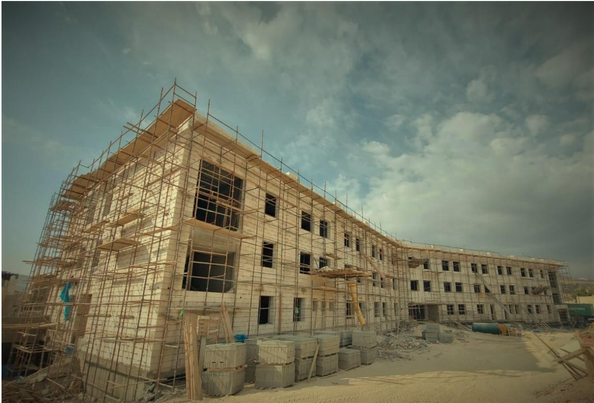
General view of the project site
