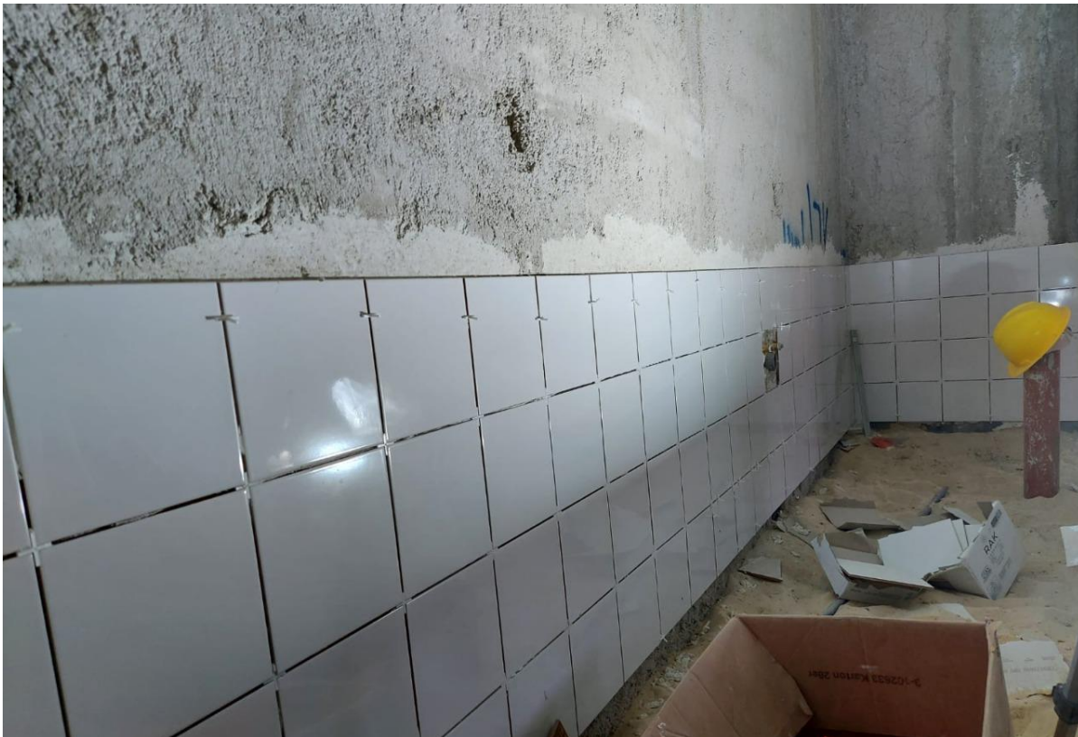
Tiles work at toilets
