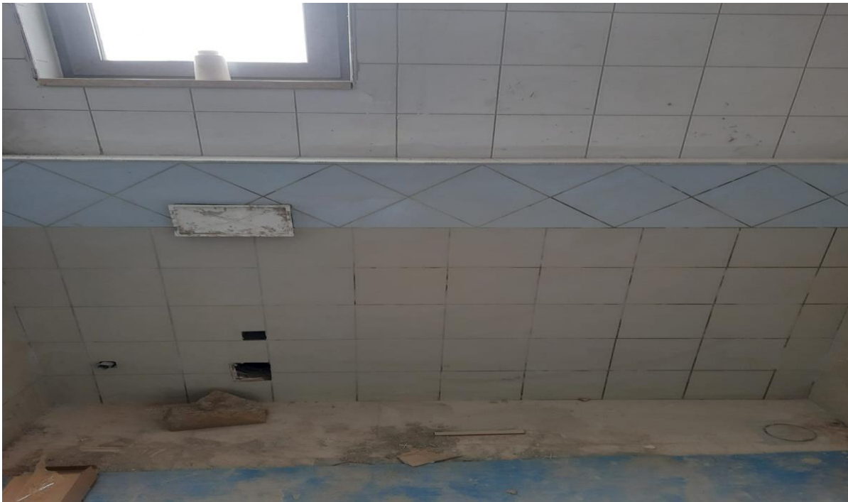
Re-tiling of wall tiles after replacing the adhesive material
