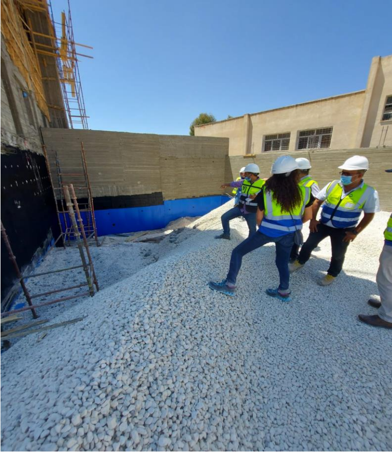
Backfilling work before completing the waterproofing layers
