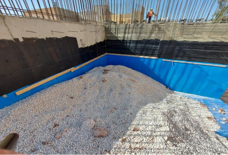
Completing the waterproofing work before backfilling
