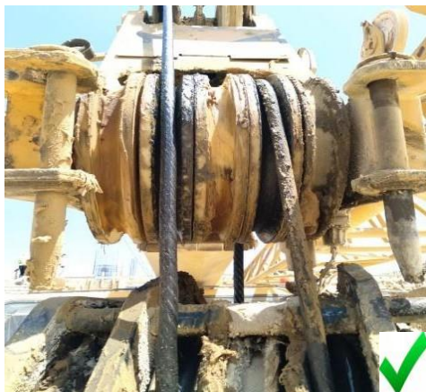
Figure (3): No Structural Issue Can be Found Here
