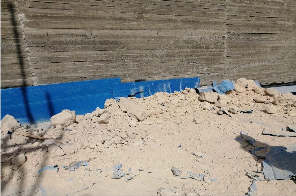
Boulders collected to be used by Contractor as backfilling material
