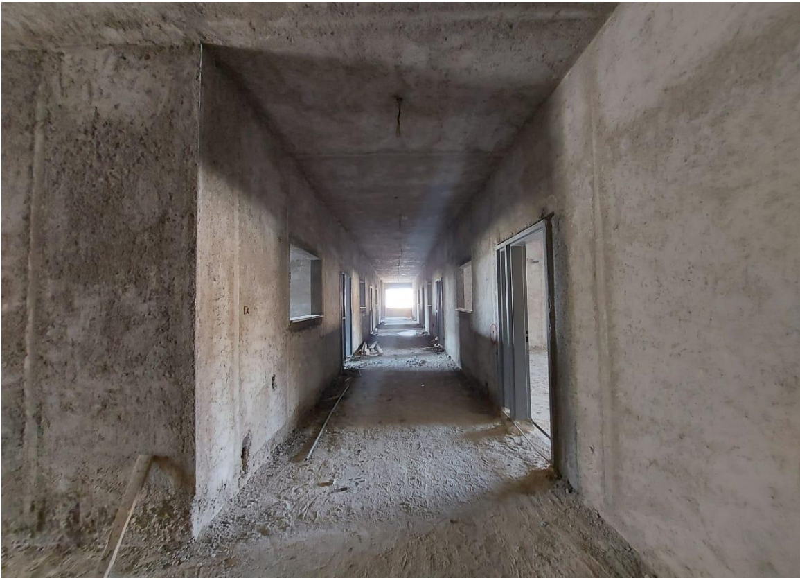
Inspecting plastering work
