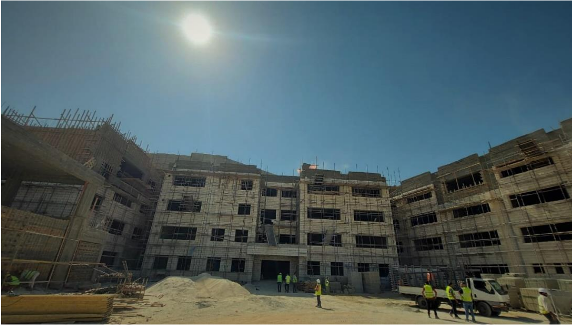
General view of the project
