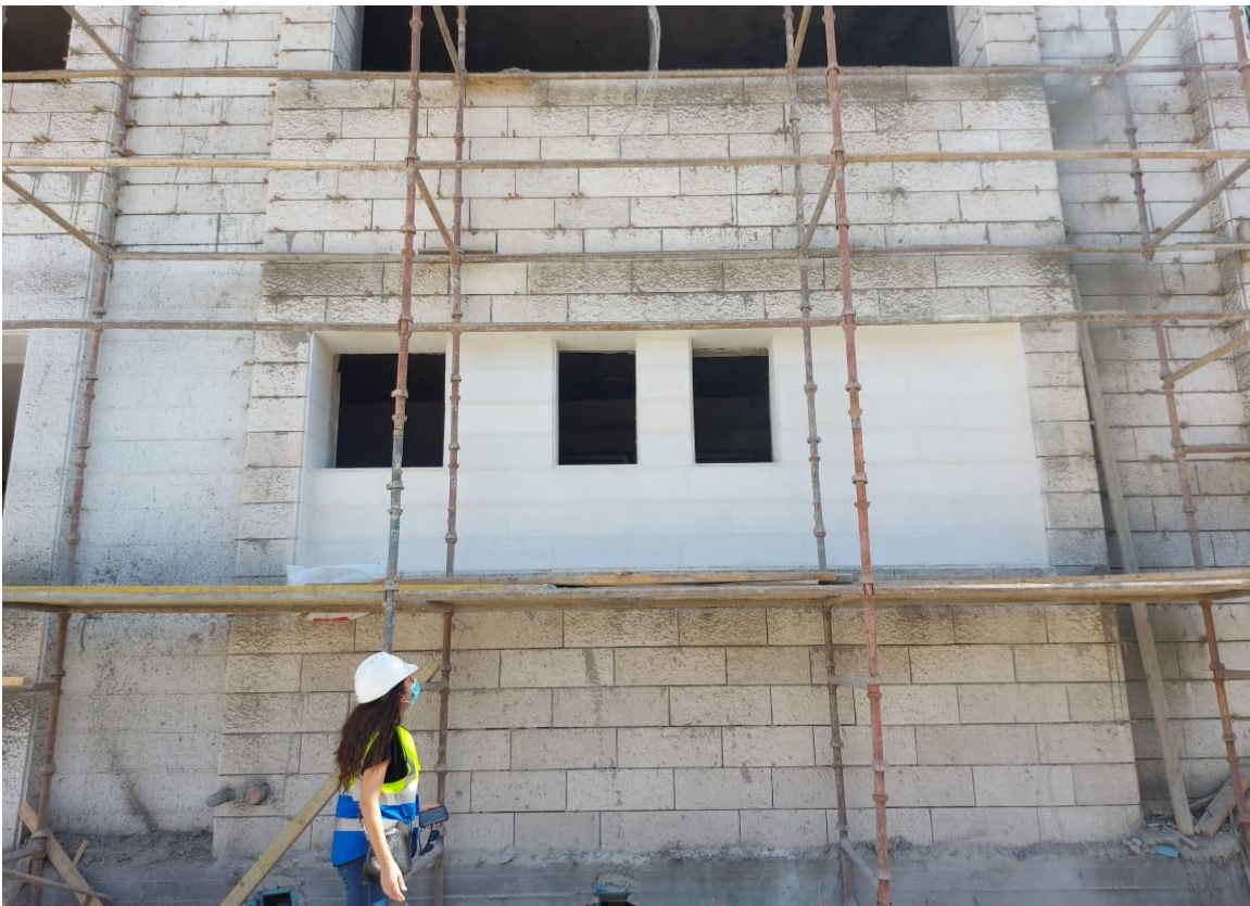
Inspecting stone pointing sample
