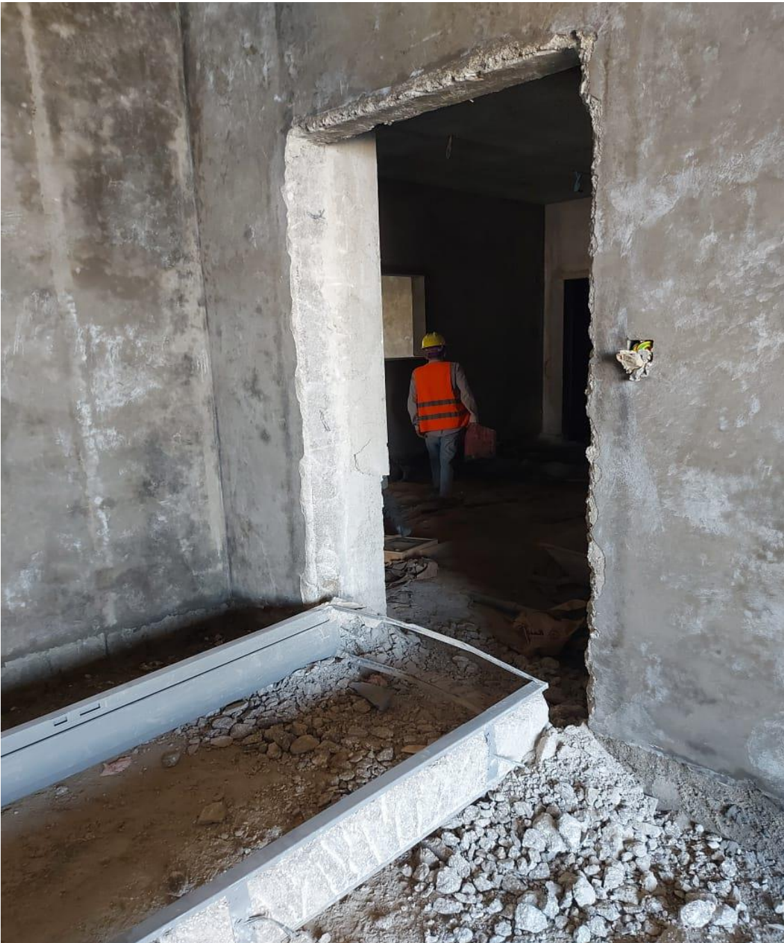
First stage of replacing defected frames
