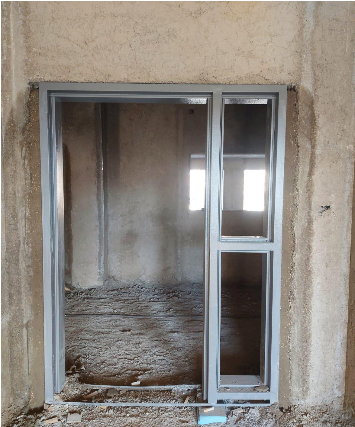
Replaced door frames with the correct dimensions
