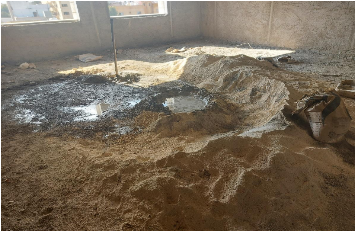
Mixing mortar without container
