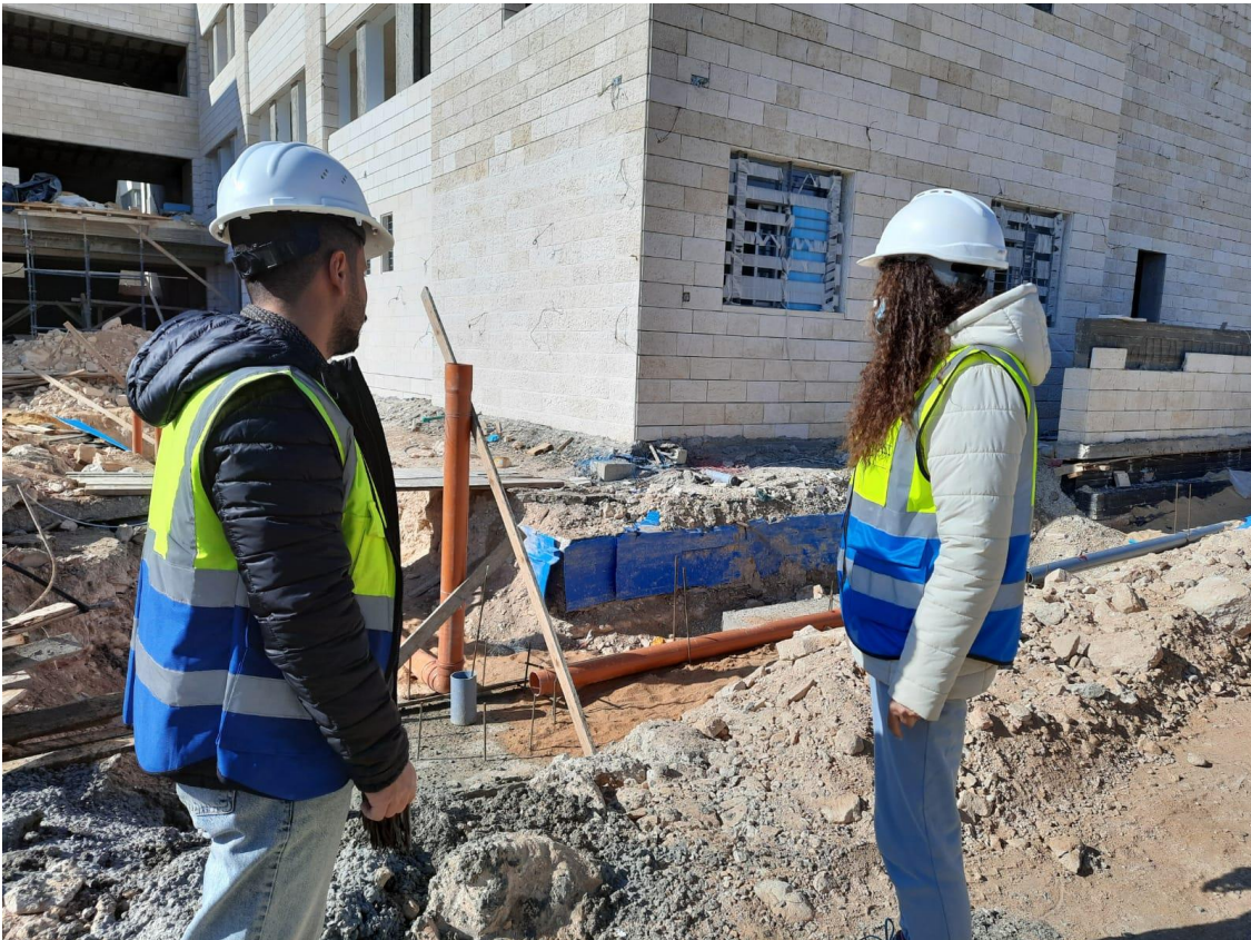
Inspecting the installation of sewer pipes
