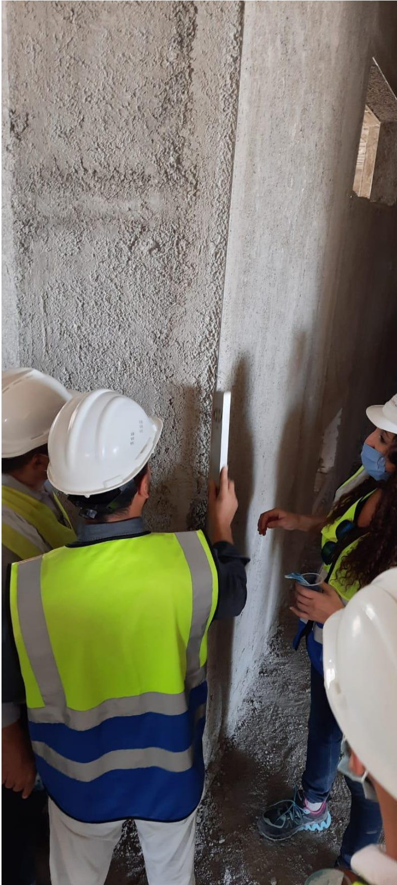
Checking the verticality of the plaster Bead
