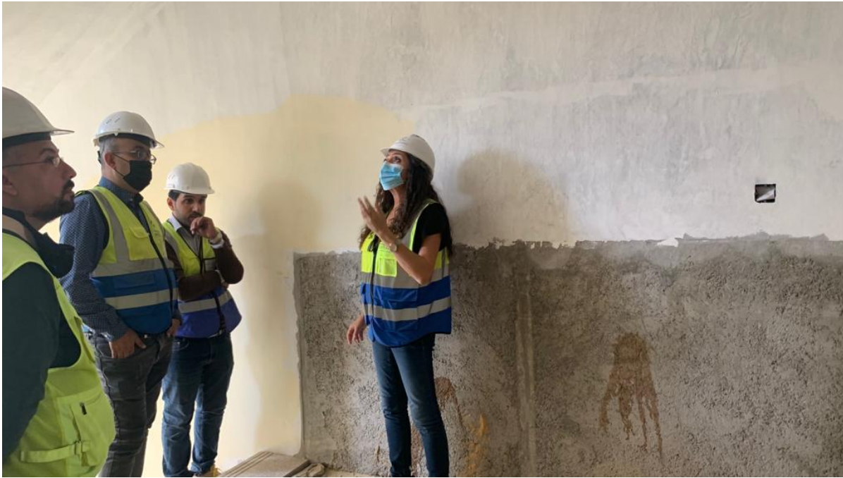
The limits between the porcelain tiles for corridors and the porcelain skirting for staircases have been discussed
