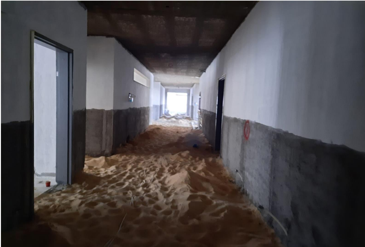
Filling materials under corridor tiles
