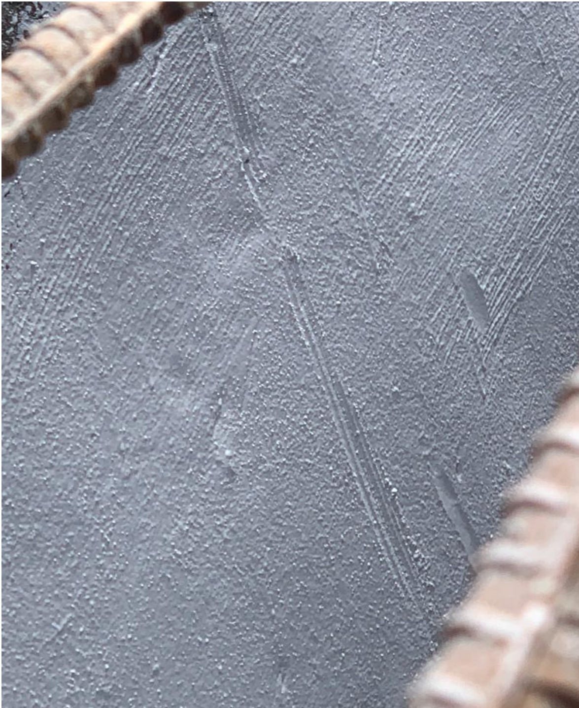
Epoxy paint for internal water tank wall
