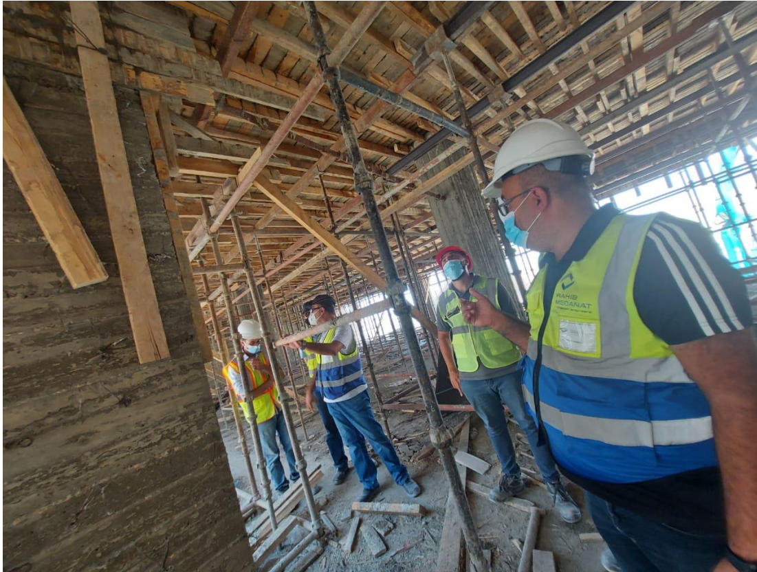
Formwork for roof slab zone "B"
