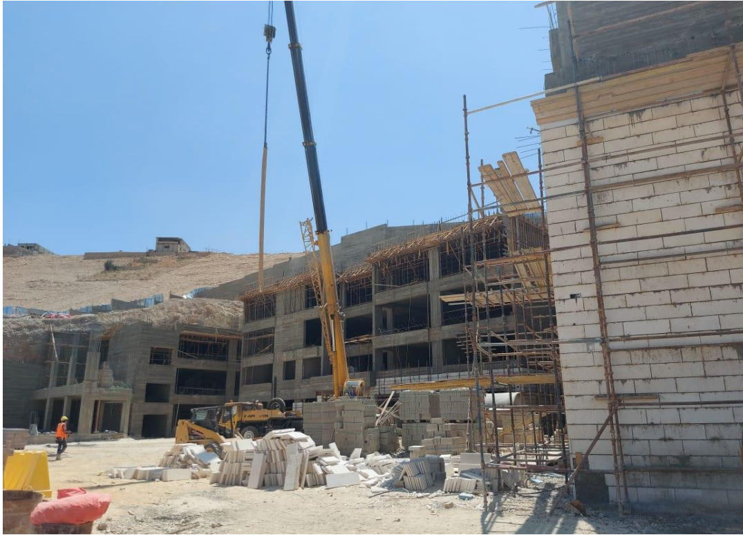
General view of the casted slab of the roof floor
