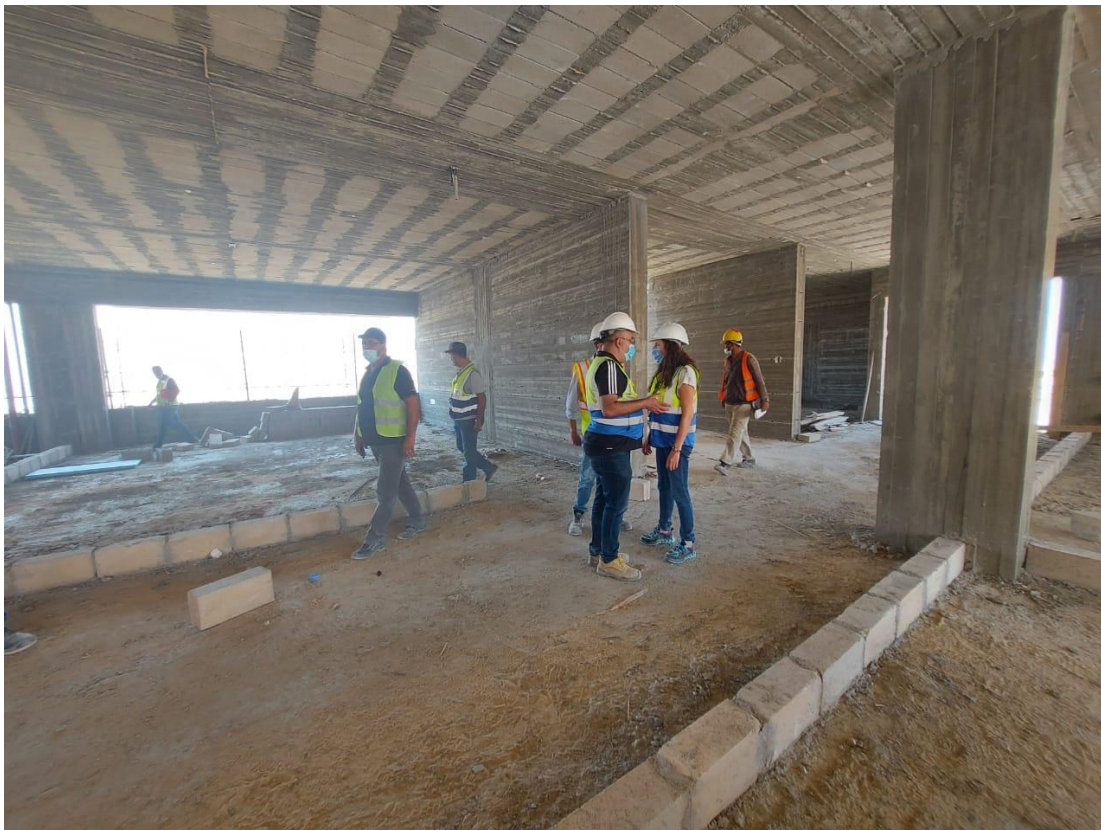
Observing first course of blockwork-second floor zone "A"
