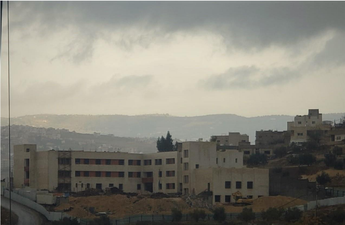
General view of the project site (Figure: 01 & 2)
