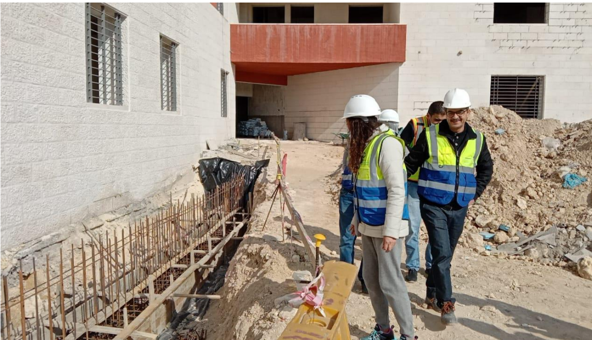
The concrete casting for external works have been inspected
