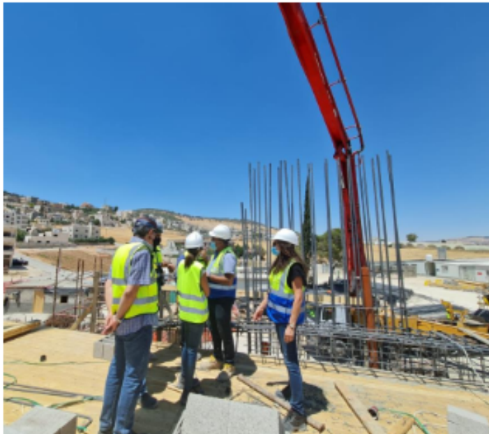
Discussing the distribution of bottom steel bars for ground floor drop beams/ground floor slab at zone A
