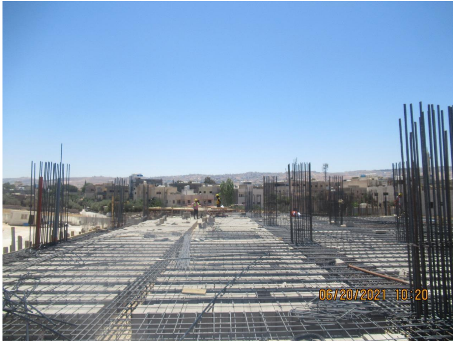
Formwork and steel reinforcement for ground floor slab Zone A
