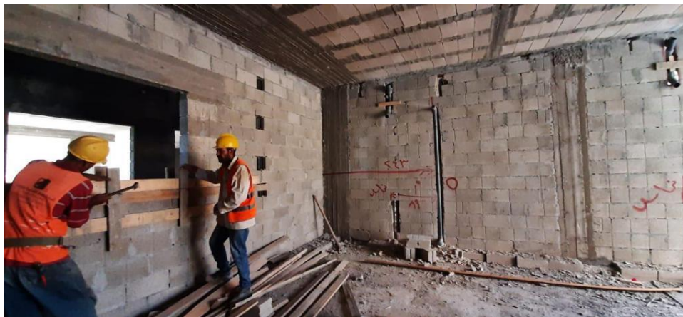
Ground floor block work zone A and mechanica l first fix
