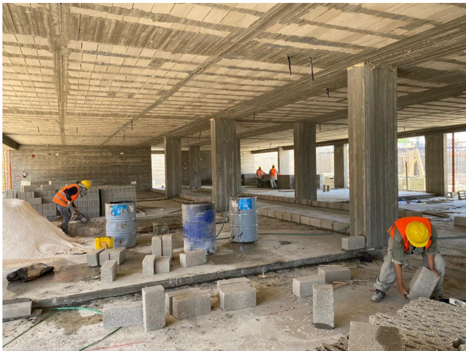
Starting Block work in the ground floor zone A
