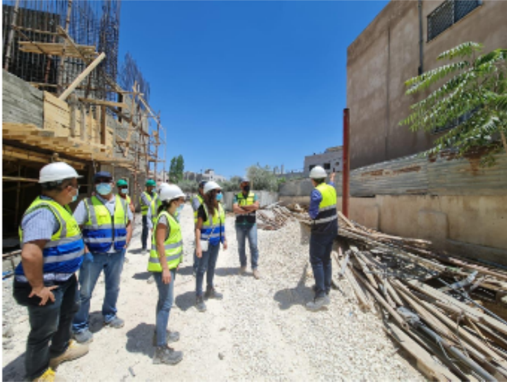
Checking the encroaching neighbor's building on the south-west side of school plot limits
