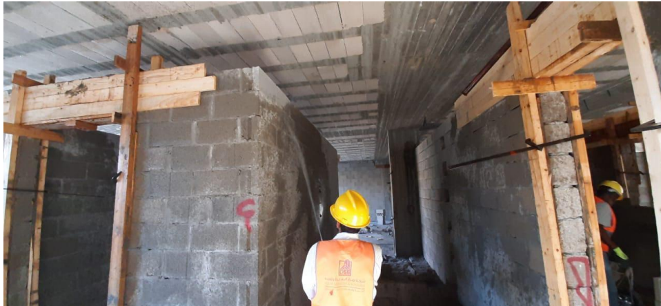
Ground floor block work zone A
