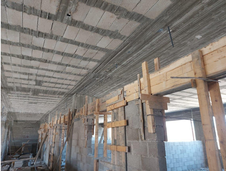
Block works for first floor at zone A of school building
