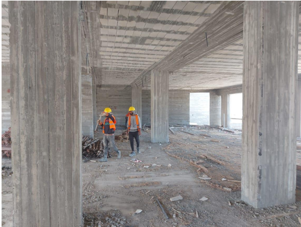
Slab formwork deshuttering
