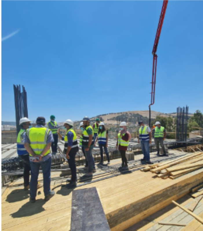
Checking reinforcement work for ground floor slab at zone A
