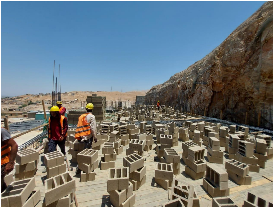
Formwork and rebar distribution for first floor slab zone C
