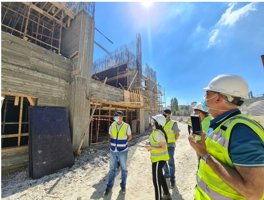
Discussing the quality of concrete walls behind stone at basement level
