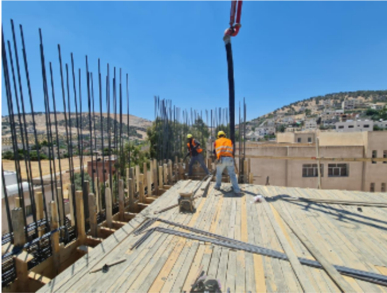
Casting last vertical element of ground floor (Core 2) at zone A
