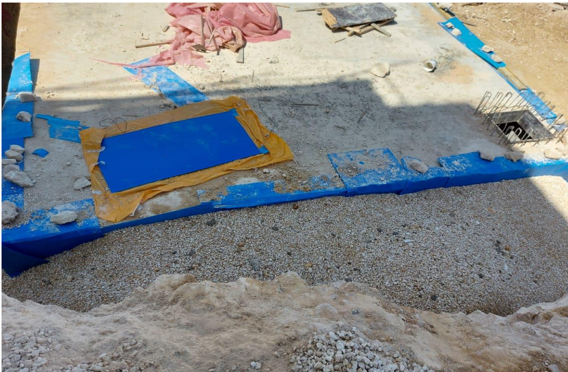
Back-filling for watertank and septic tank
