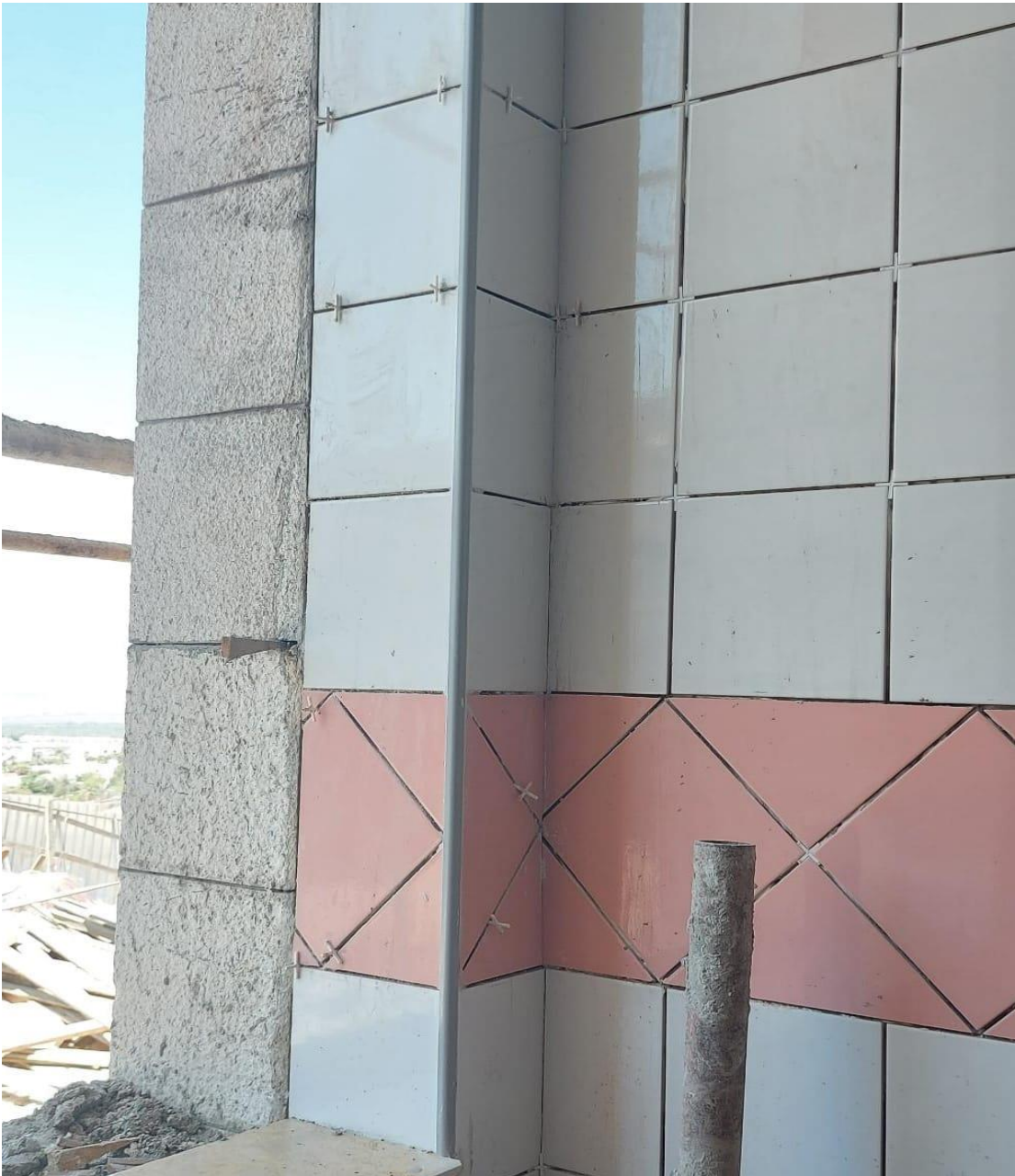
Installing corner beads for tiling works
