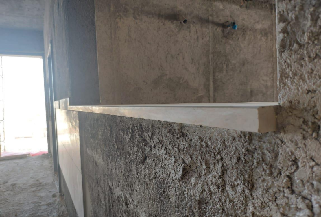
Complied sill at the right level installed
