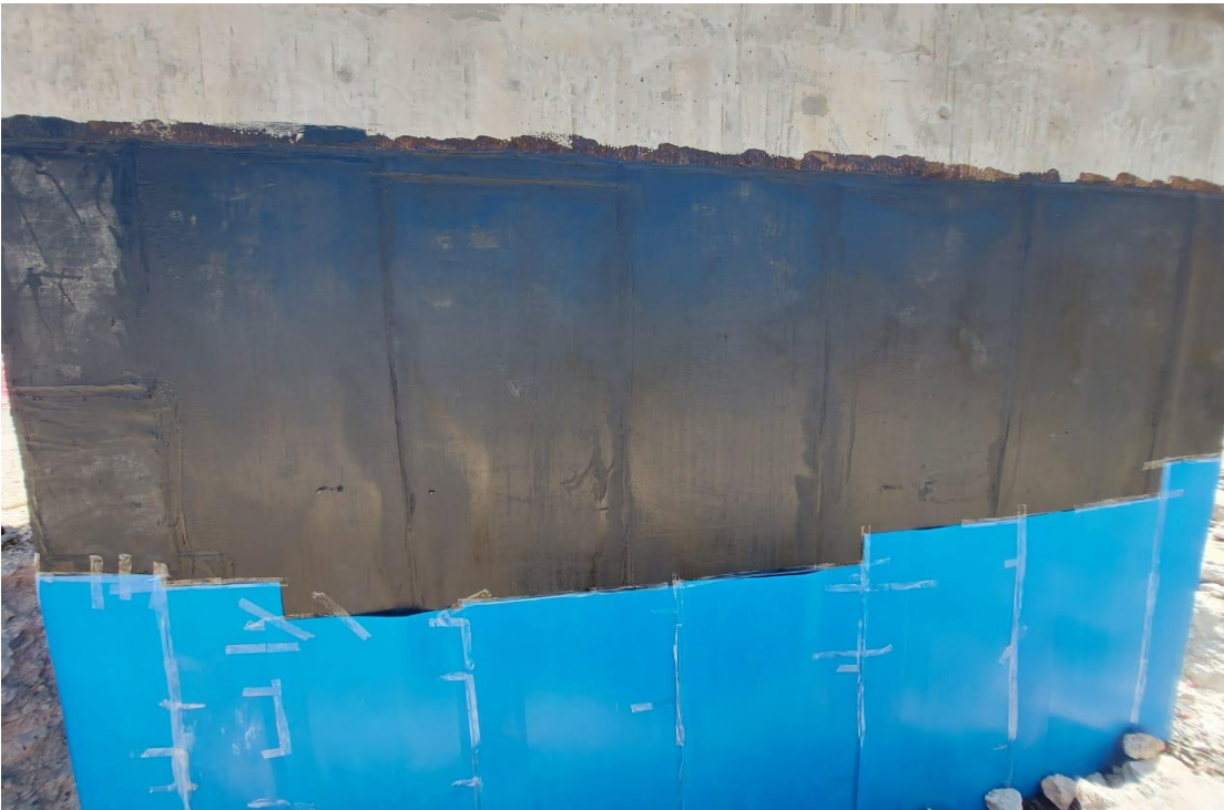
Protection for waterproofing for watertank and septic tank
