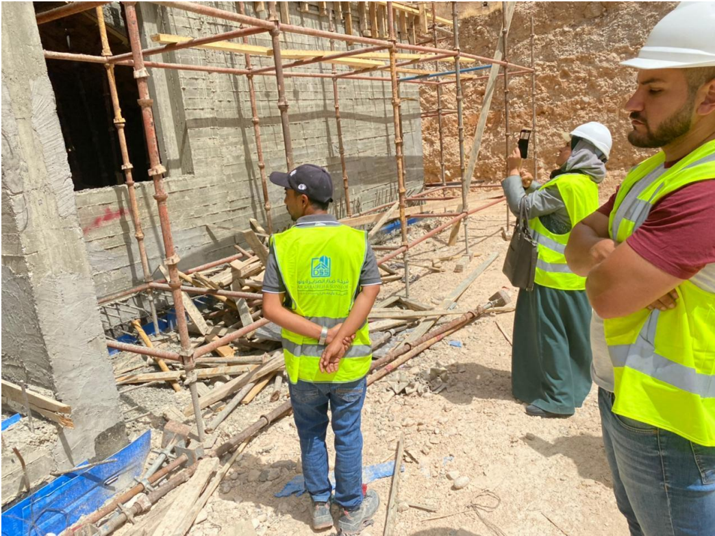
Inspecting work progress.
