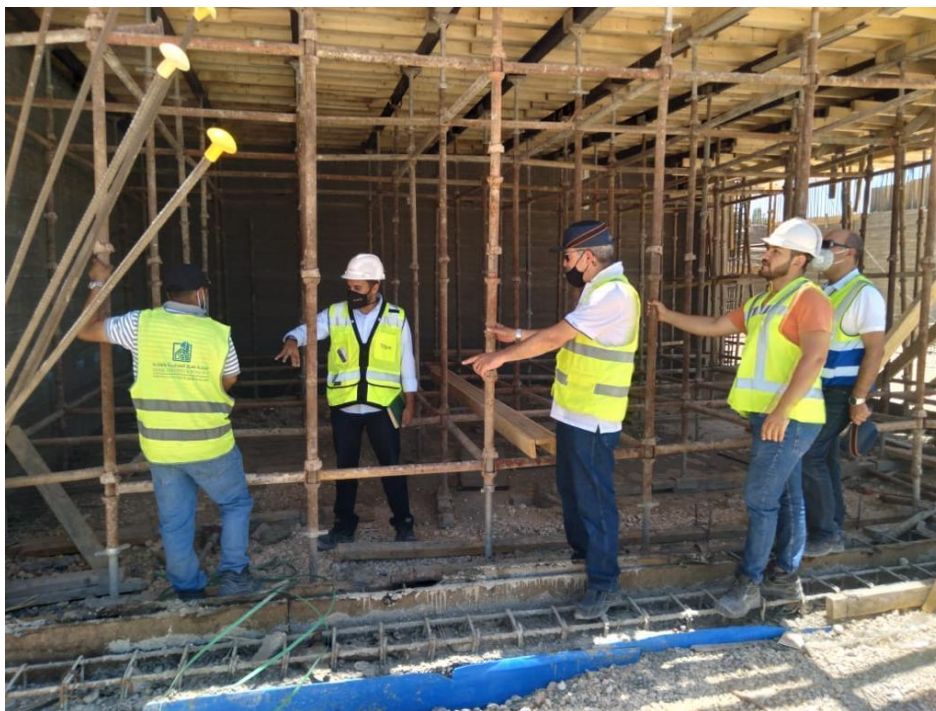
Checking ground floor columns alignment
