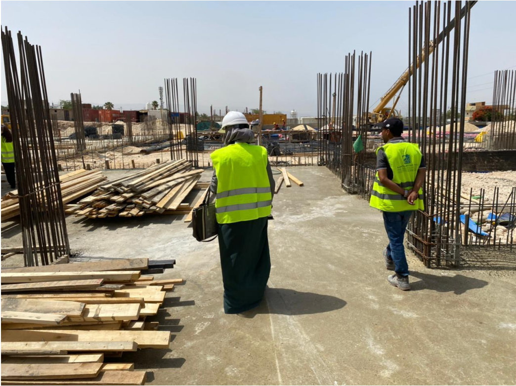
A tour inside the construction site
