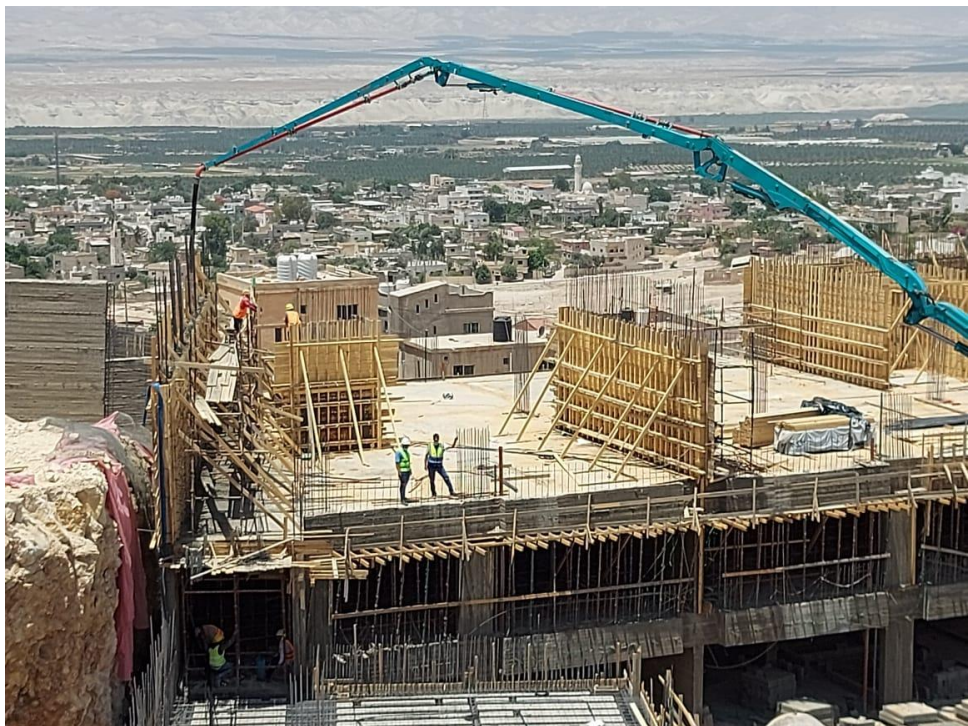
General View of the project
