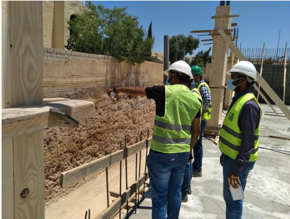
Discussing site obstacle (encroaching neighbor's wall)
