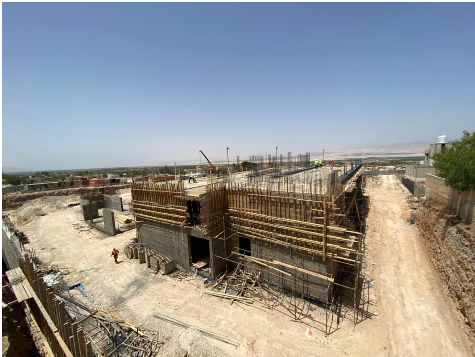
General View of the Project
