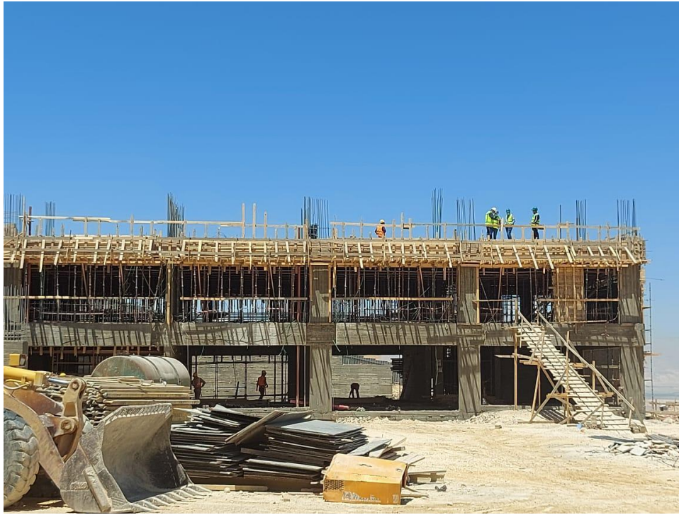
Formwork and steel reinforcement for second floor slab zone A
