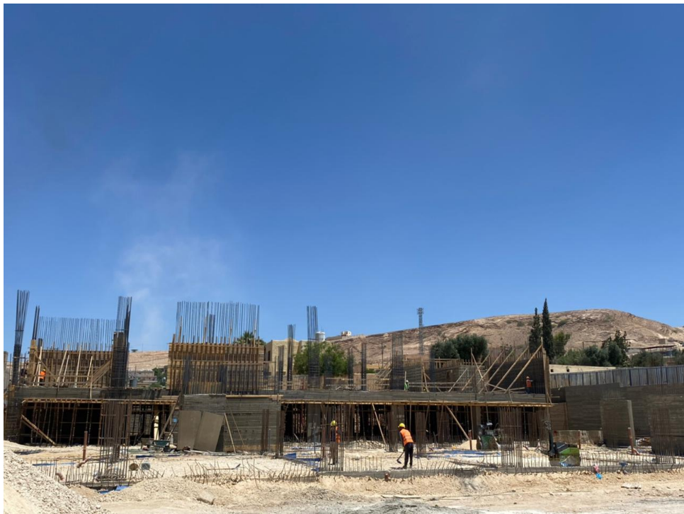
Steel reinforcement and formwork for the first floor columns and walls
