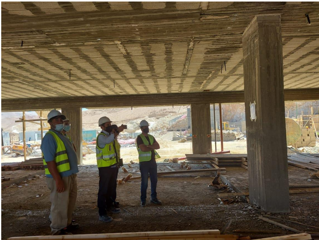
De- Shuttering formwork for ground floor slab zone (A)
