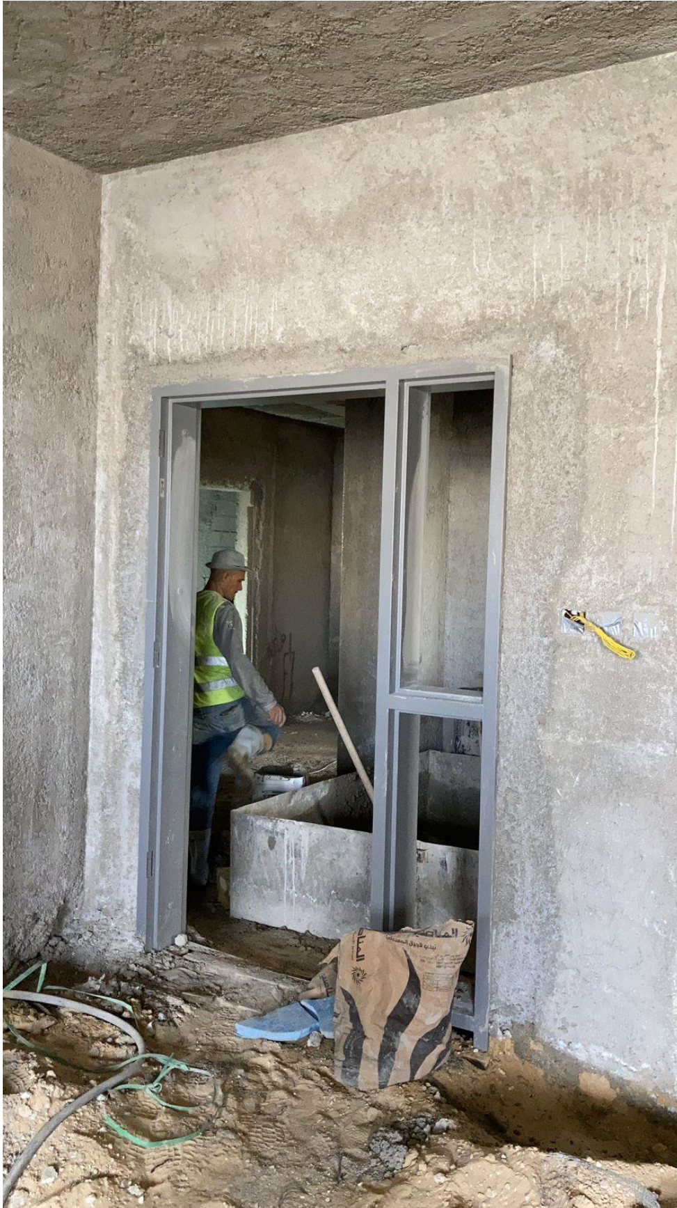
The Contractor using a container for mixing mortar for plastering
