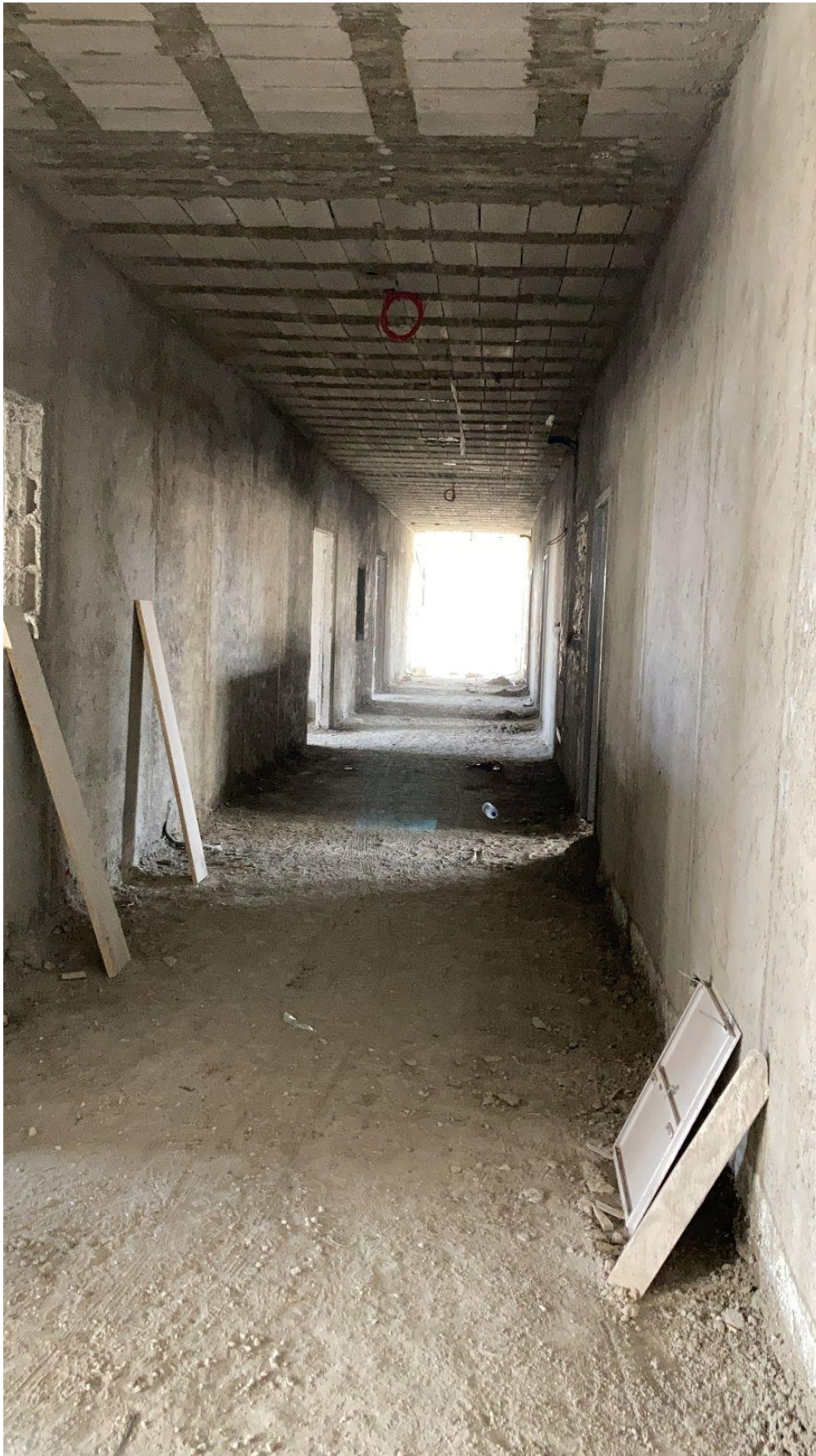
A view for the corridor showing the executed plaster work
