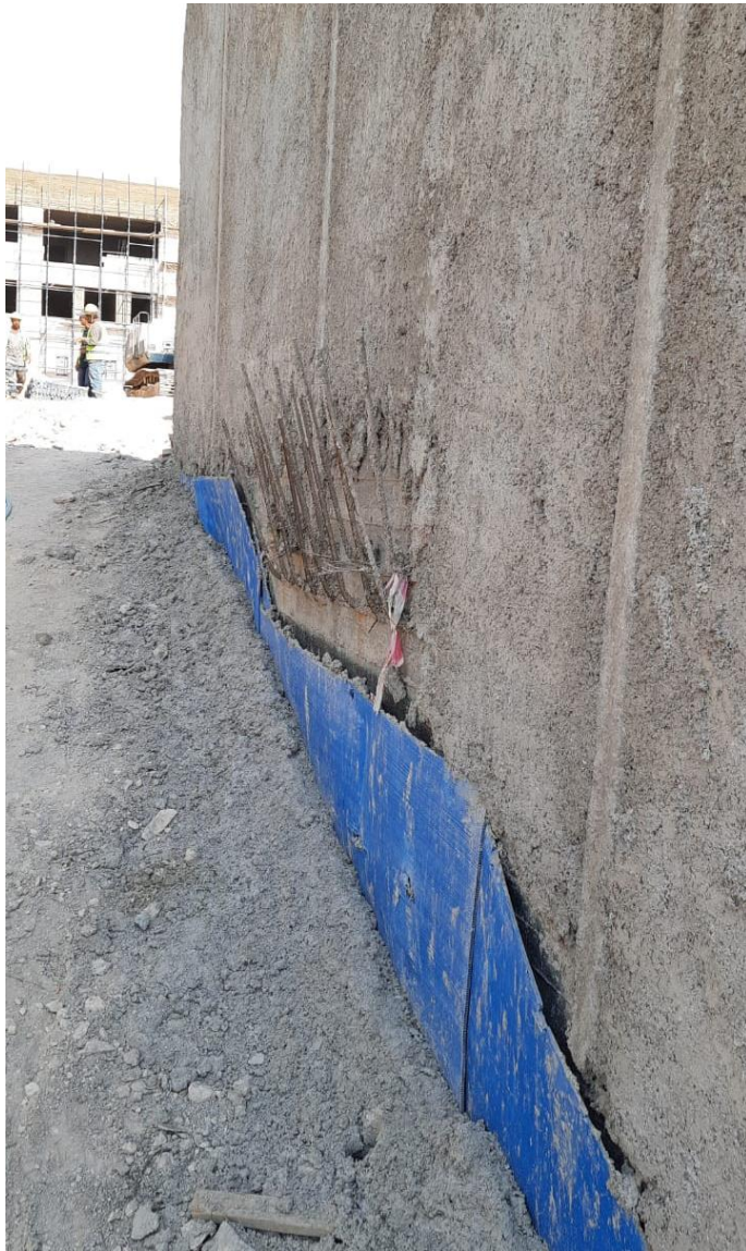
Before applying safety caps on reinforcement steel bars
