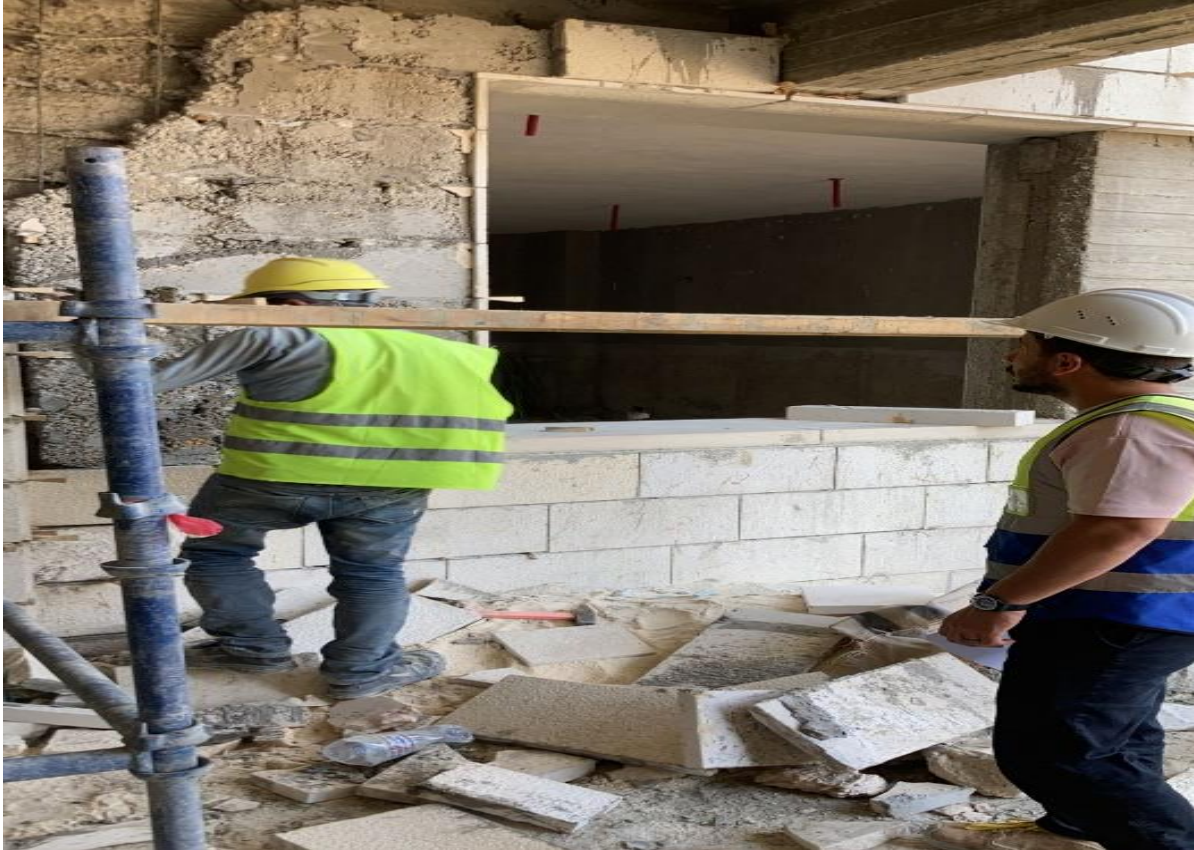
Removal of defected built stone
