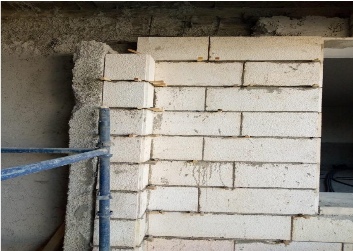
Re-building the stone correctly
