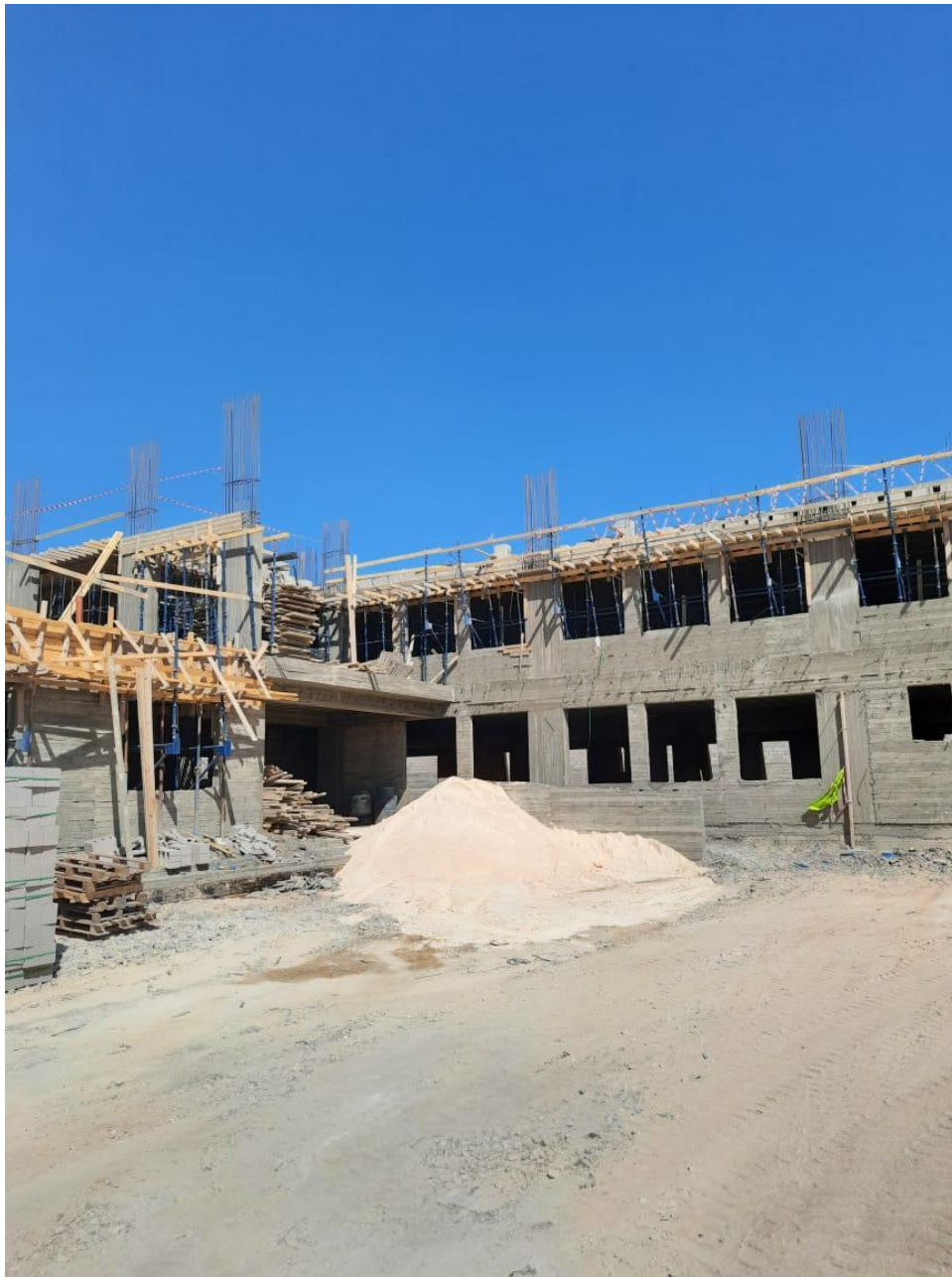
Formwork for the first floor slab part 1
