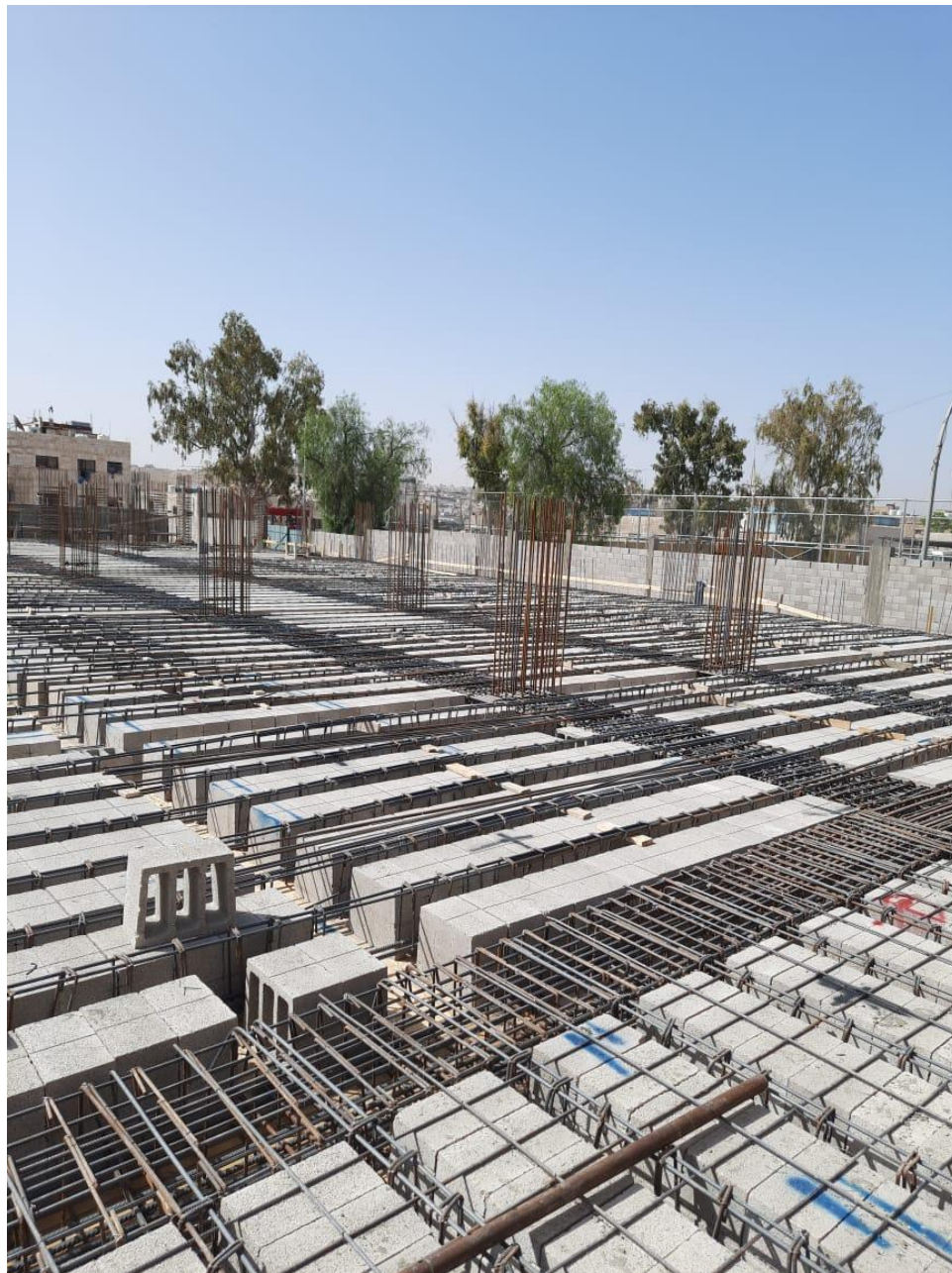
Steel reinforcement for ground floor slab part 2
