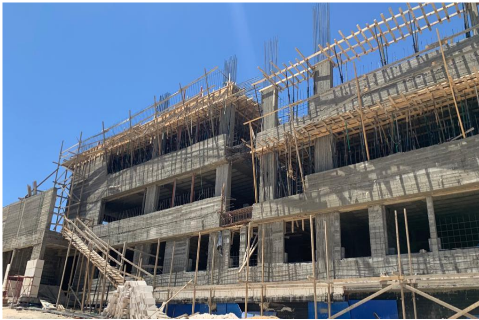
formwork for second floor slab - part 2
