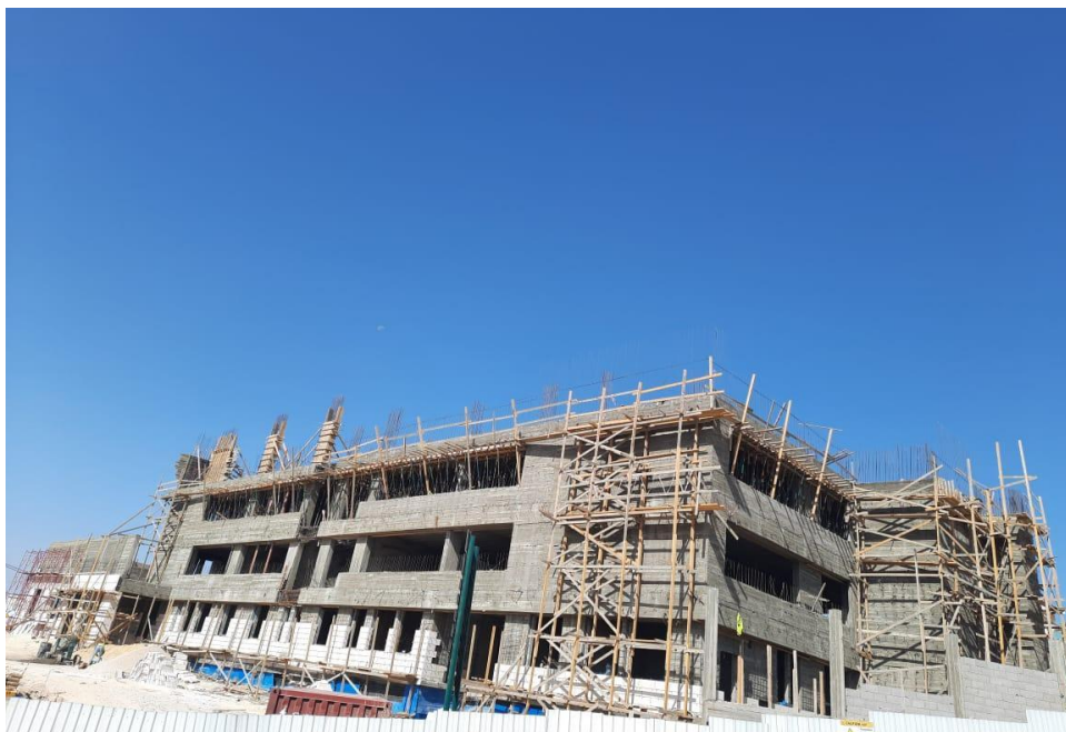
General View of Project site
