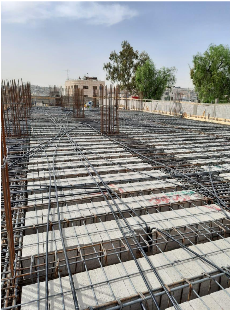
Steel reinforcement and electrical pipes first fix
