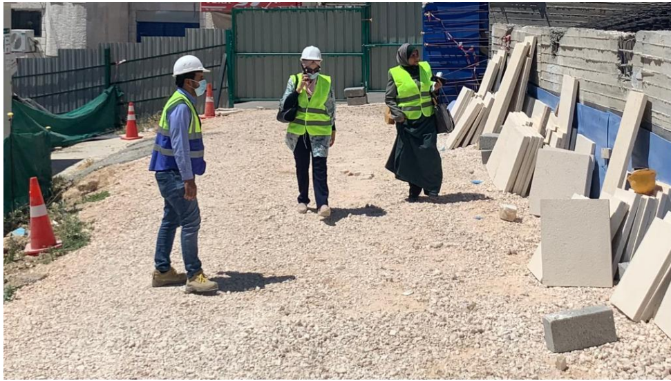
Tour around the site was conducted
