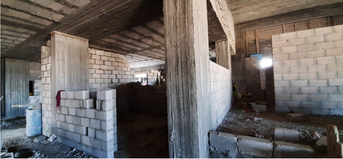
Inspecting blockwork at the multi-purpose hall/ground floor
