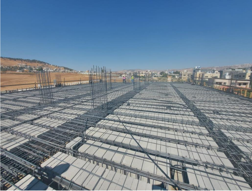
The first floor roof slab at (Zone B) is under preparation
