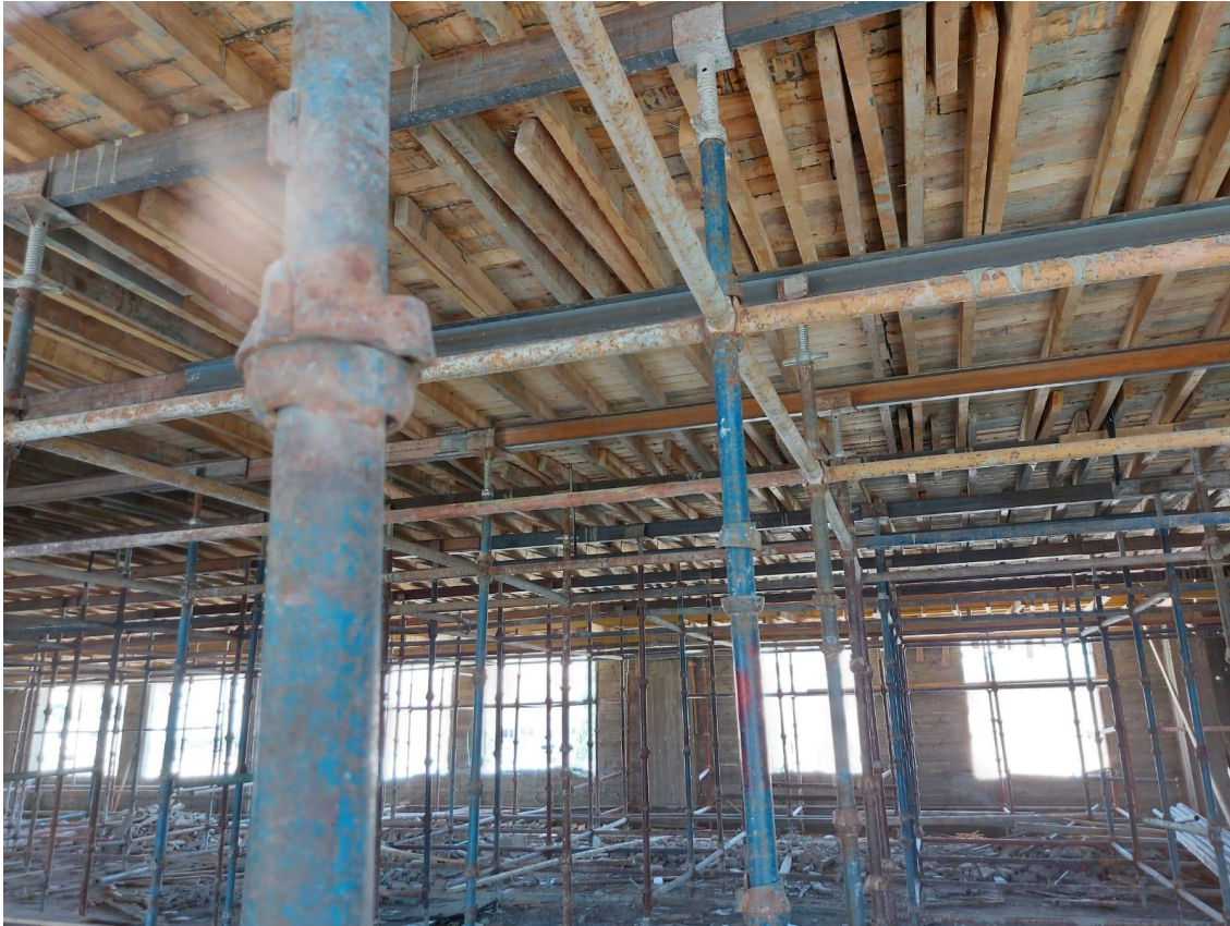
Scaffolding and formwork for second floor slab zone "B"
