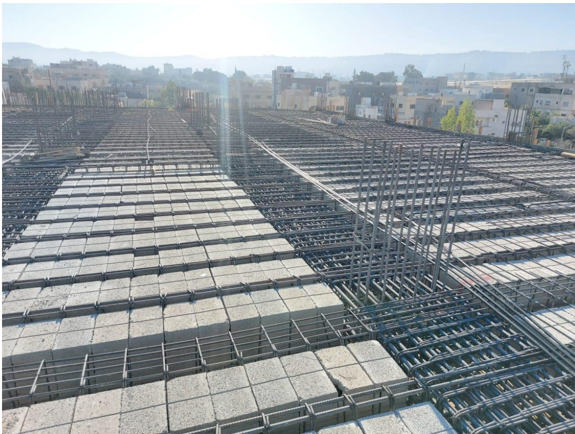
Reinforcement work at second floor slab zone "B"
