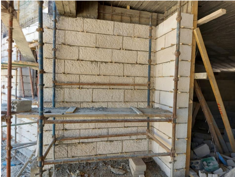
Stone work for School main entrance
