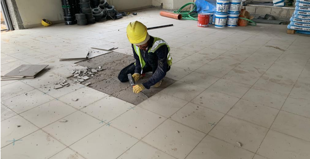
Starting with the removal of defected porcelain floor tiles
