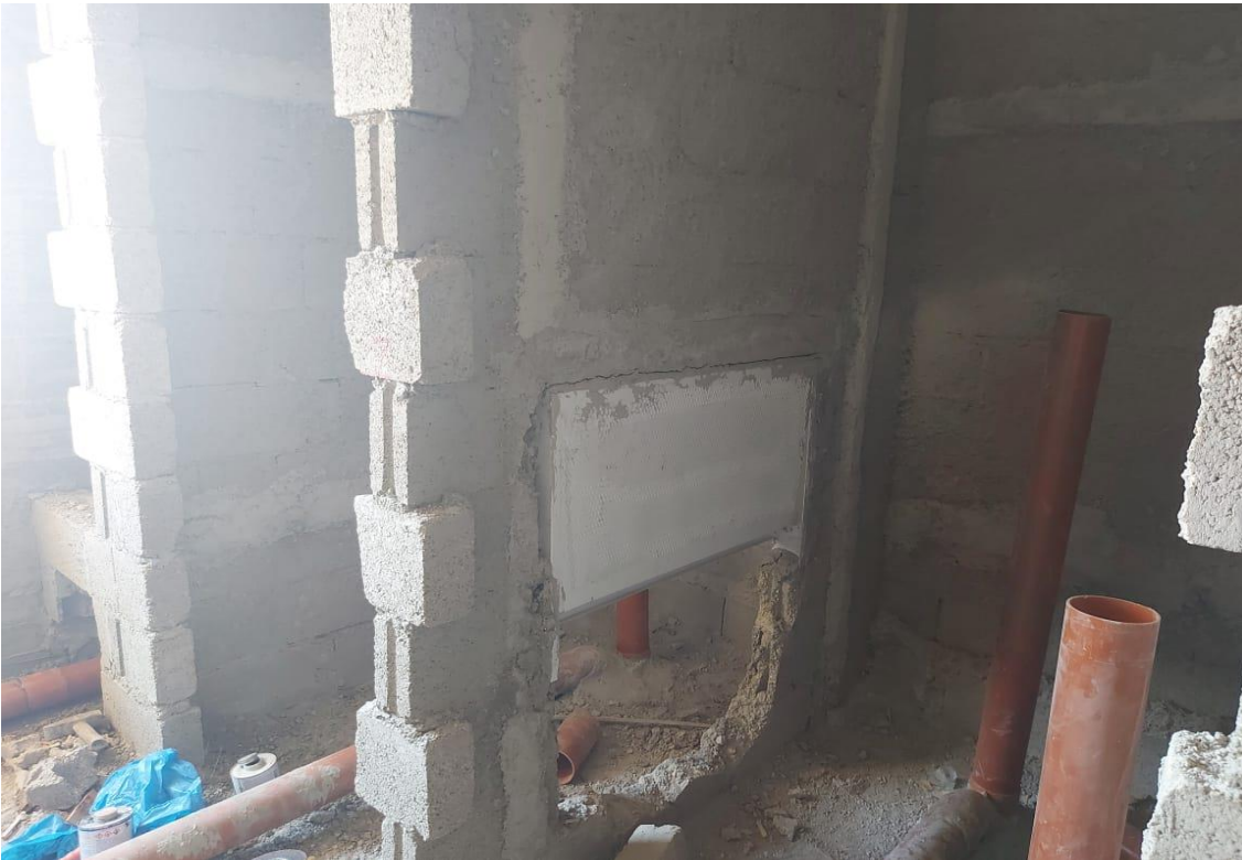
Case of Mechanical Cabinets installation
