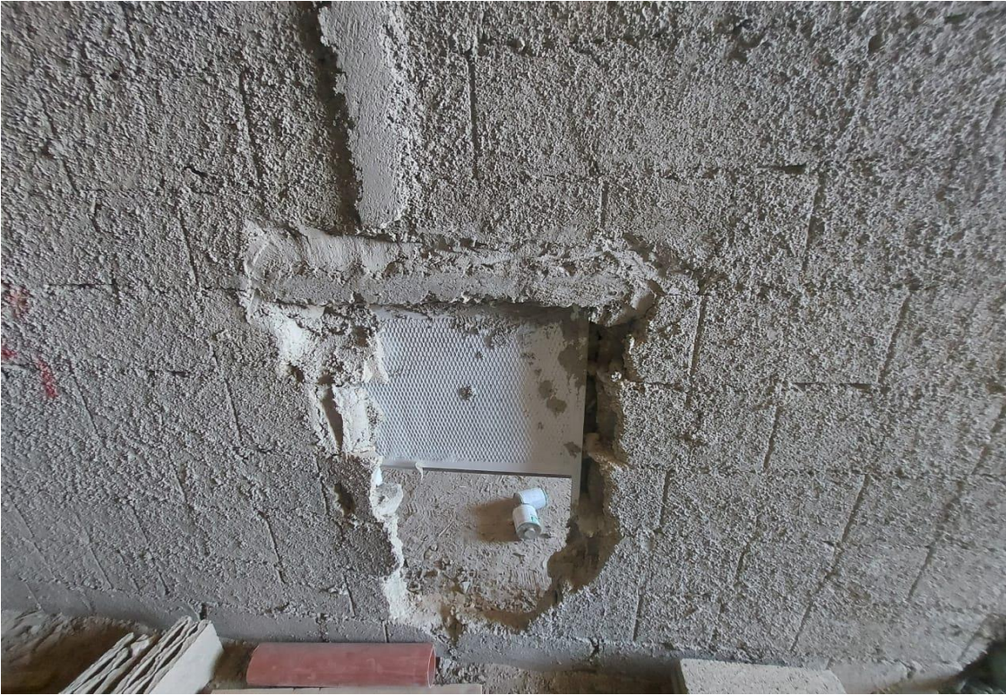
Starting to rectify Mechanical Cabinets Installation
