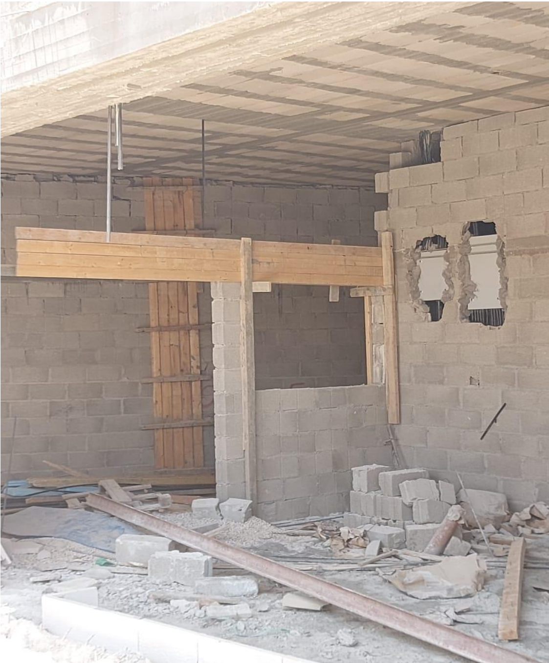
Mechanical Cabinets Installation
