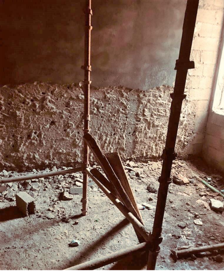
Removing of final layer of plastering
