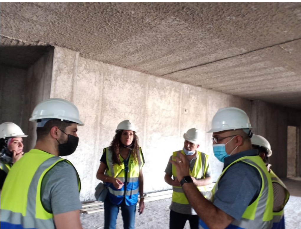
Observing plastering work and remarks were given
