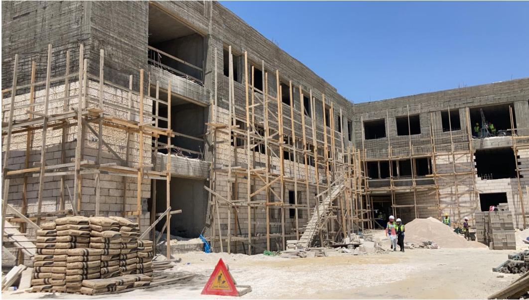
General view of the completed second floor casting (the last slab)
