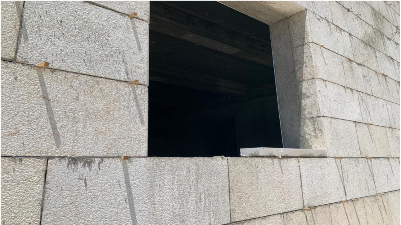
Replacing stones
