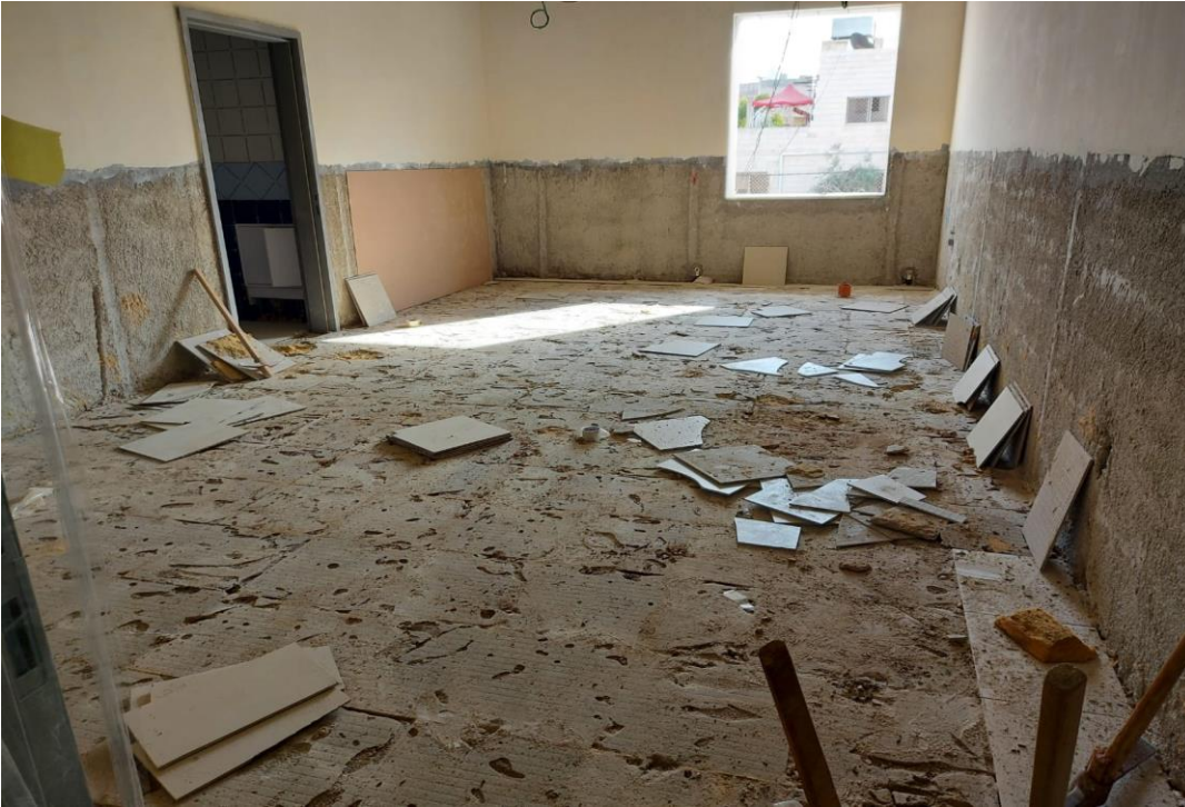
Removal of defected porcelian floor tiles
