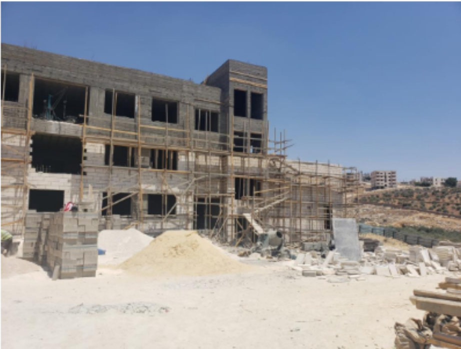
The Contractor is continuing in removing the defected stones to replace them with stones complying with the approved sample. Special zone at the site was identified to sort out the stones and discard the rejected stones. Stone building is still progressing
