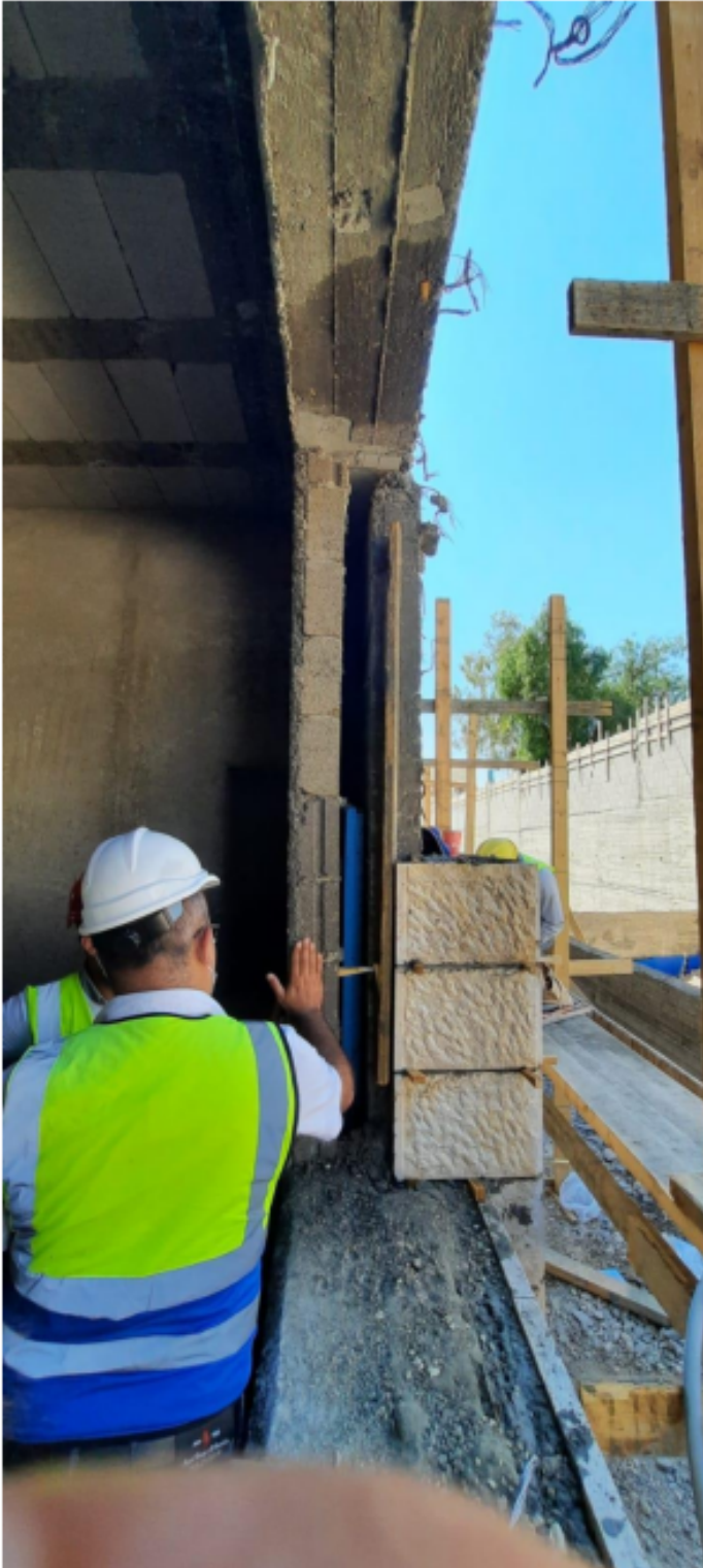
Eng Natheer explaining the correct way to execute window jambs formwork
