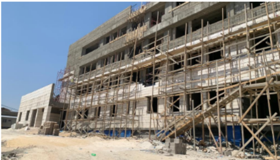
General view of the completed third floor casting (the last slab)
