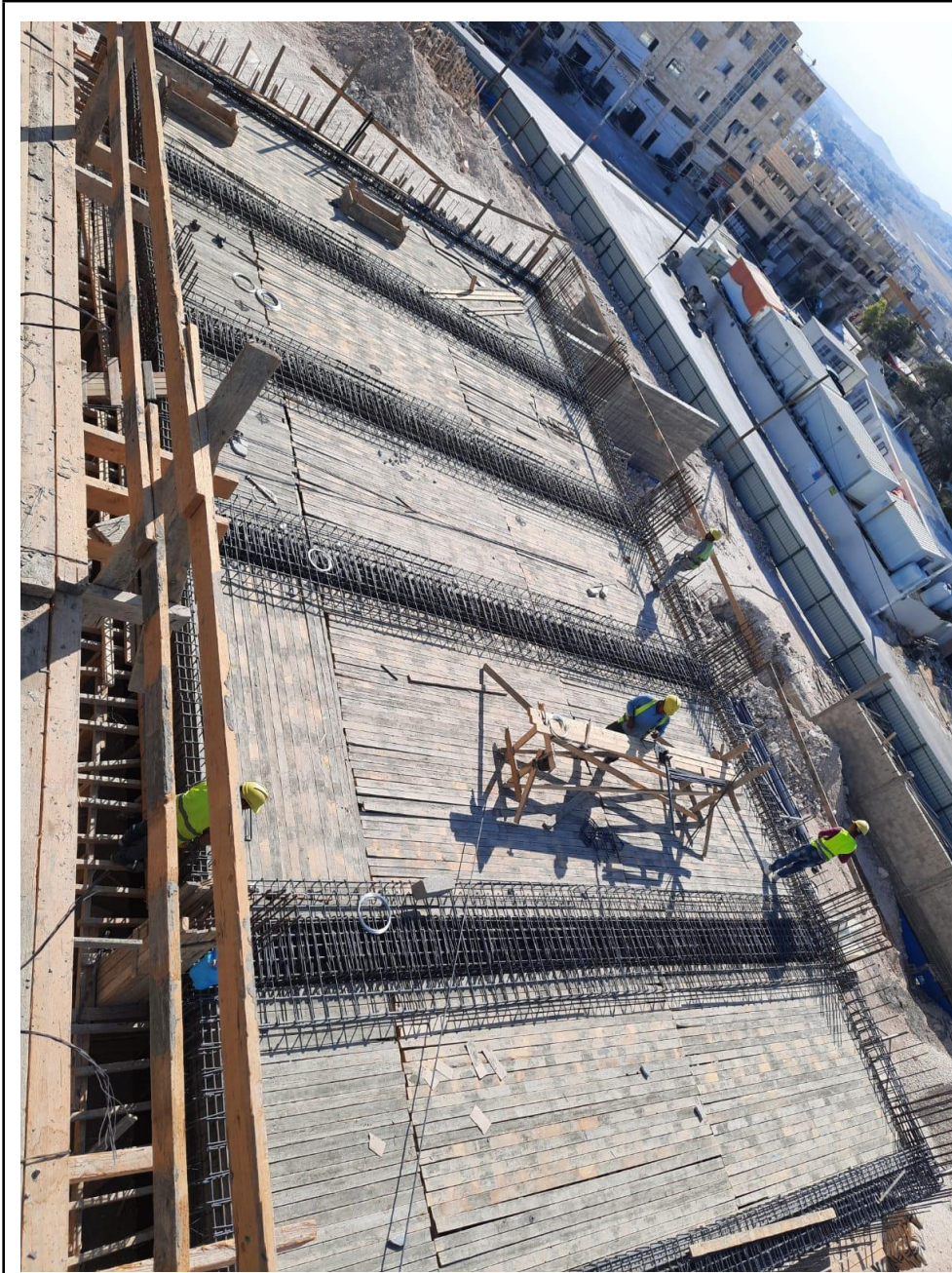
Formwork for the theater slab
