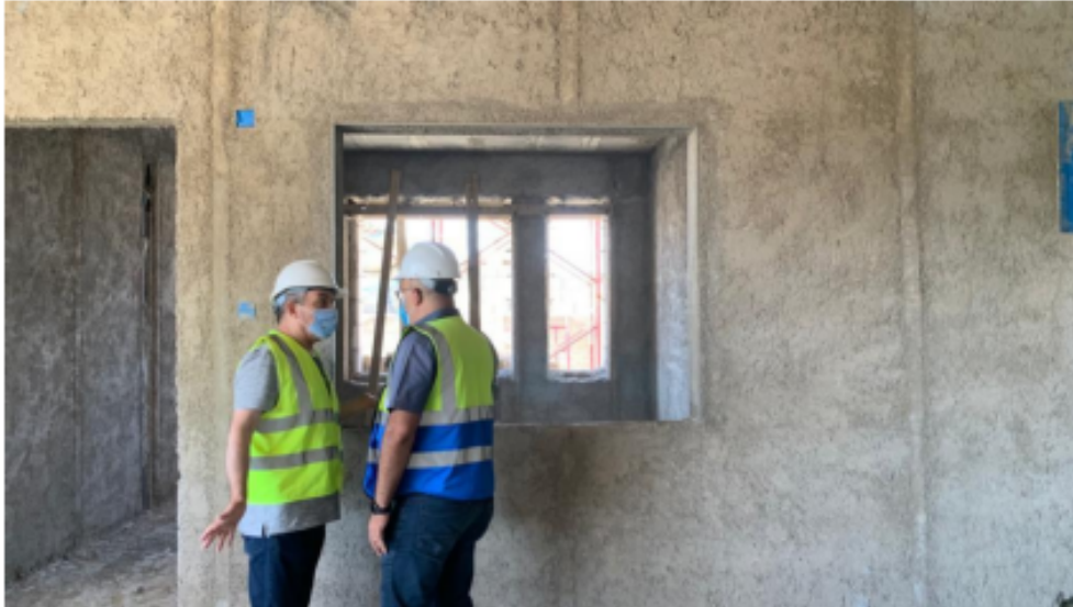
Plastering beads are used for windows' edges
