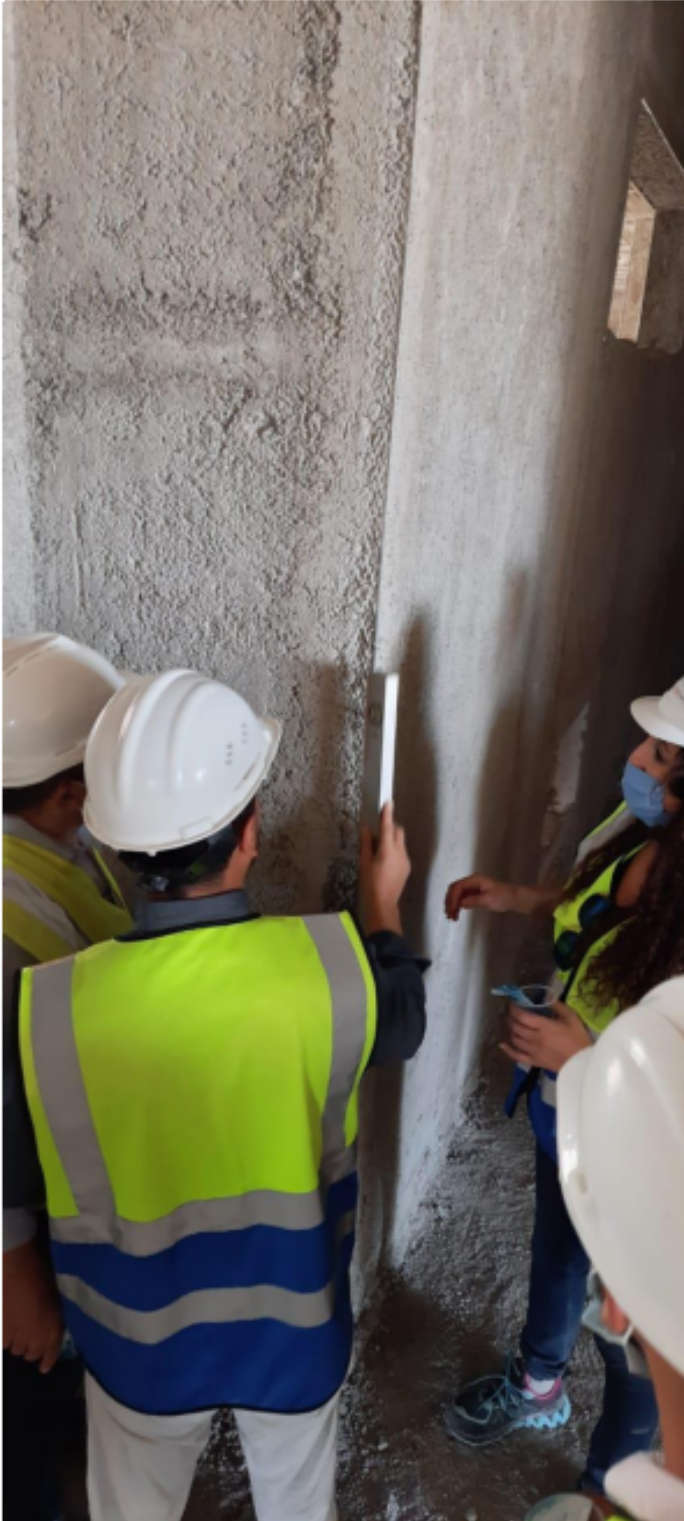
Checking the verticality of the plaster Bead
