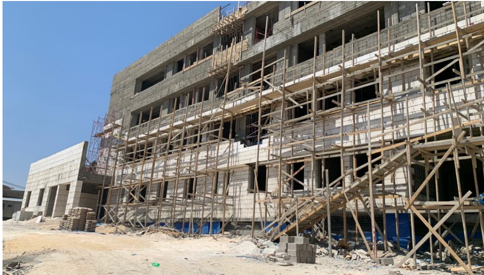
Stone cladding at the eastern elevation
