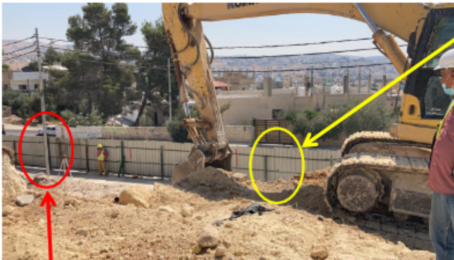
-Relocating the temporary fence adjacent to the encroaching street
