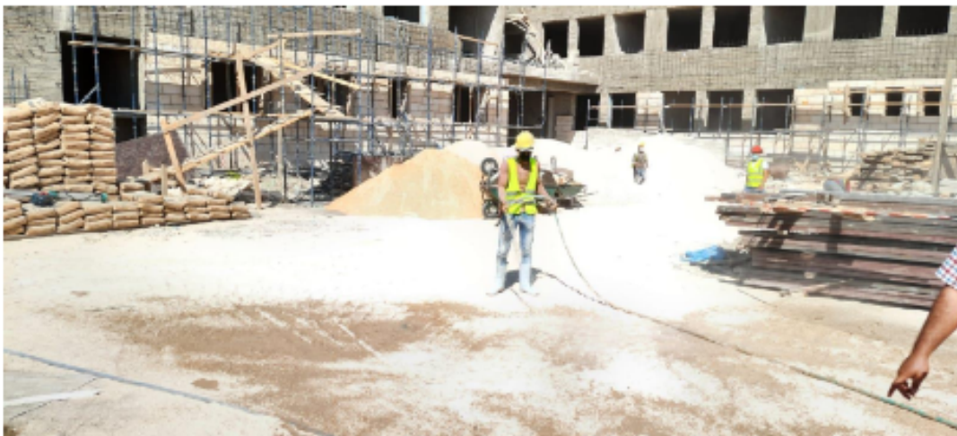
Spraying water at the sand areas in the site for the purpose of dust control
