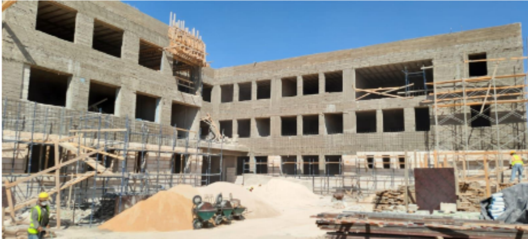
General view of the completed roof floor casting (the last slab)
