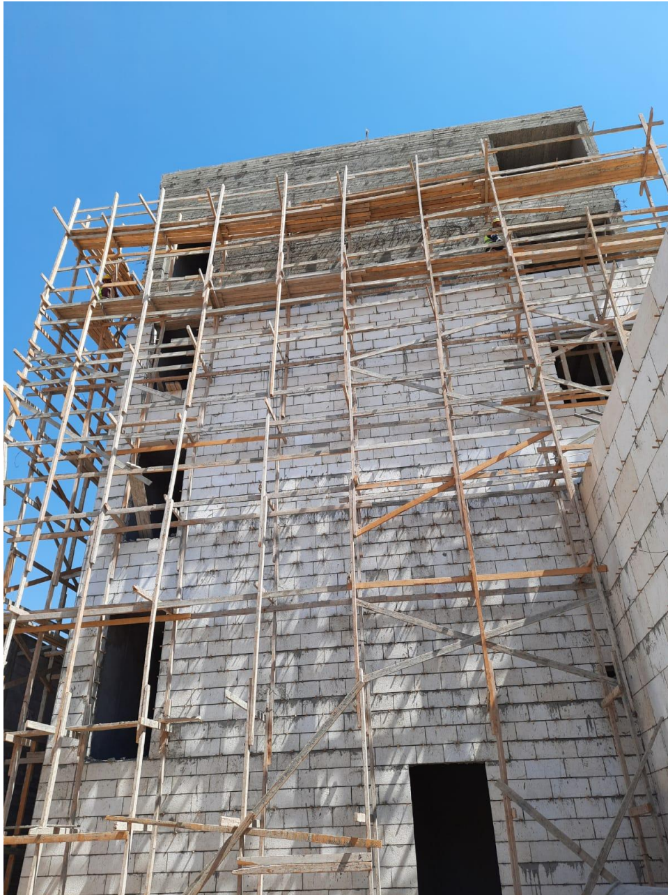
Stone Cladding at the southern elevation
