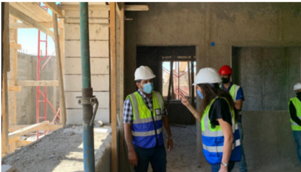
Discussing connection between backing concrete behind stone and window jamb with the internal finishing
