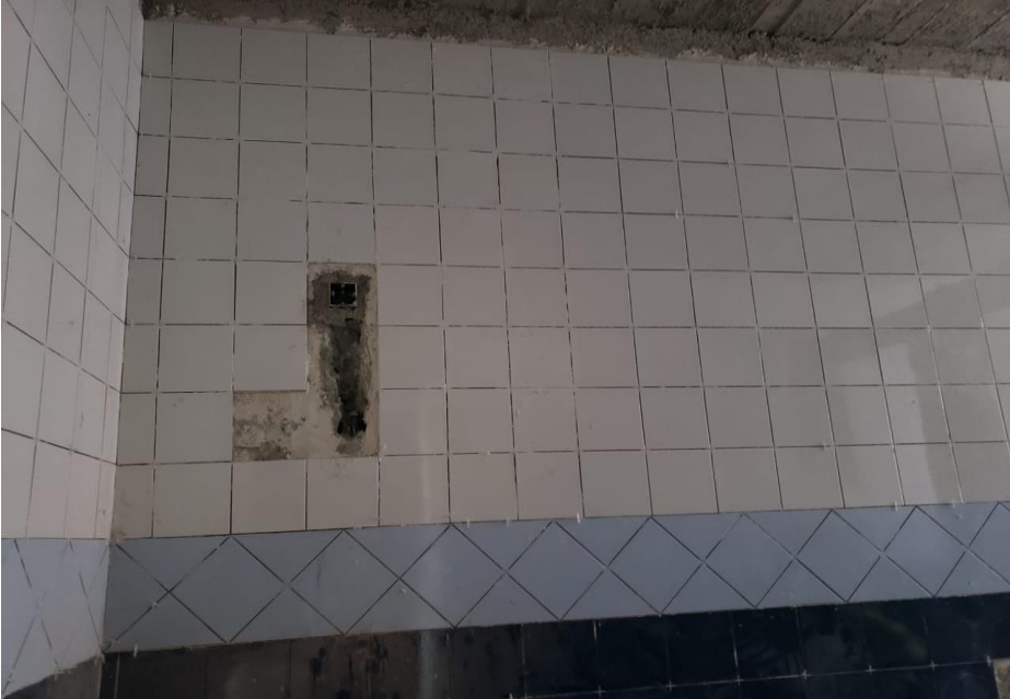
Retiled wall in accordance to the shop drawings
