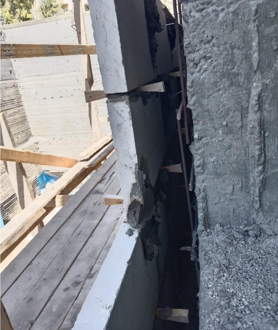
Wooden wedges within backing concrete space
