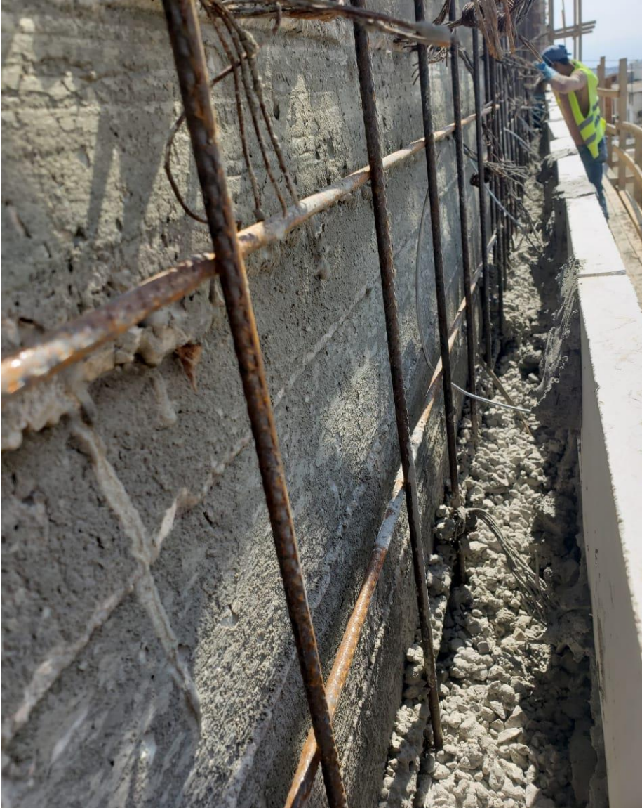
Removing wedges out of the backing concrete space
