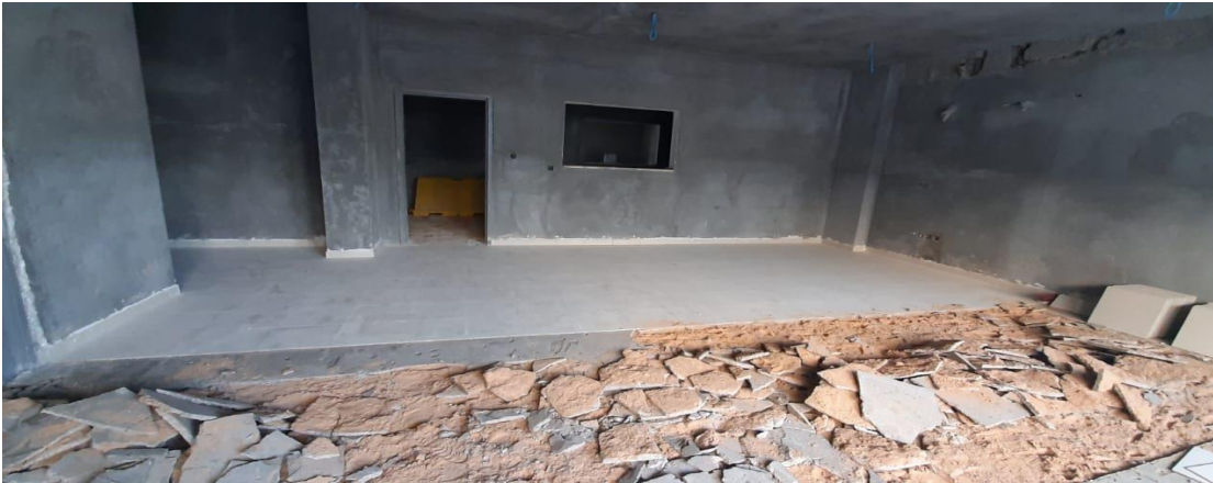
Starting with the removal of defected porcelain floor tiles
