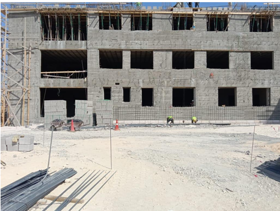
Starting the stone work (first row)
