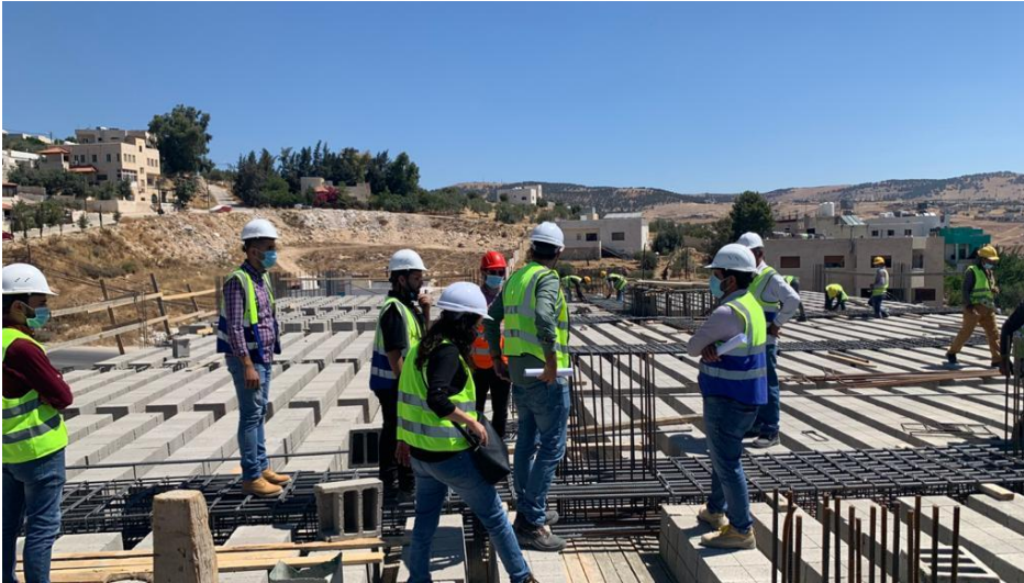
Top of Second floor's slab
