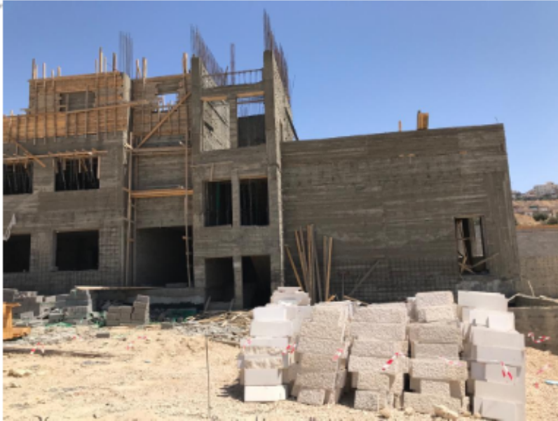
← Steel Reinforcement of part B of the First floor slab and curing works for the casted part A
