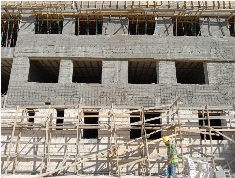
Progress in stone works and finishing the final slab- part 2
