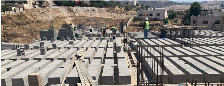
Formwork and steel reinforcement for 3rd floor slab- part 2
