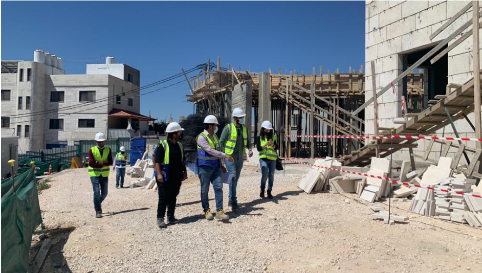
Tour inside the site was conducted
