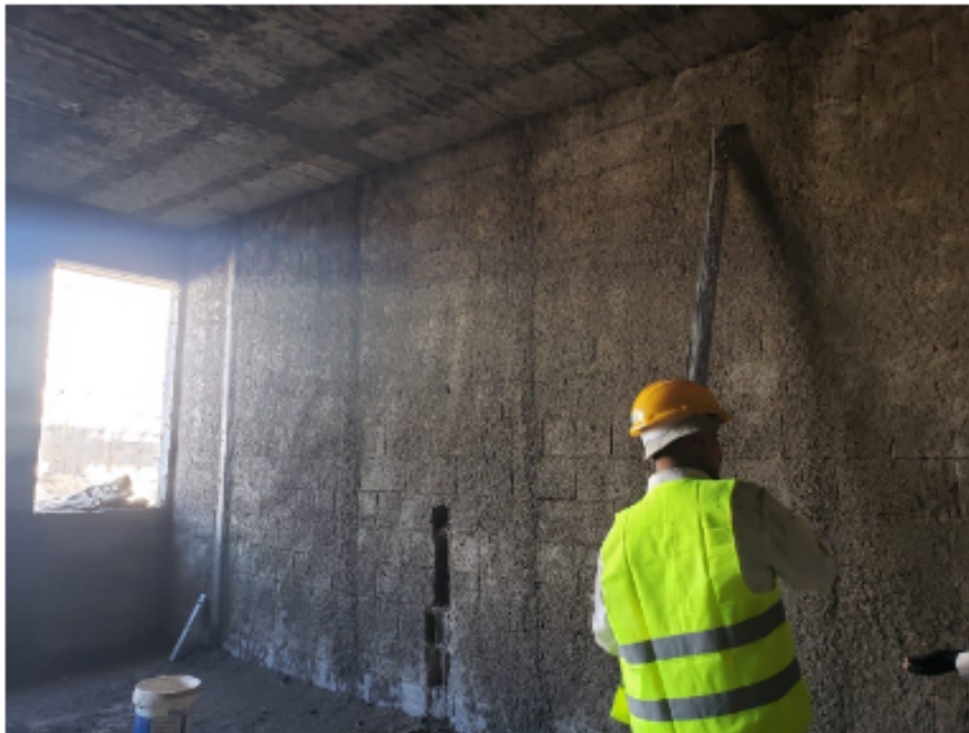
First stage of plastering work
