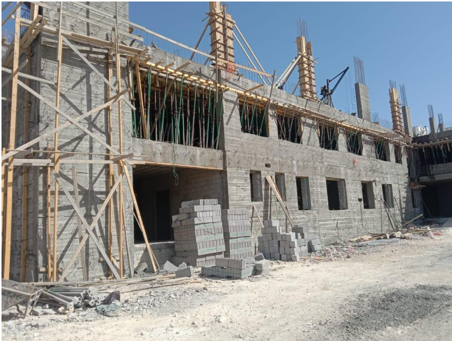
Columns formwork for the second floor)
