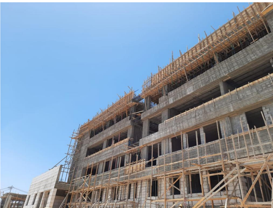
Shows the progress of stone work and finishing the final slab
