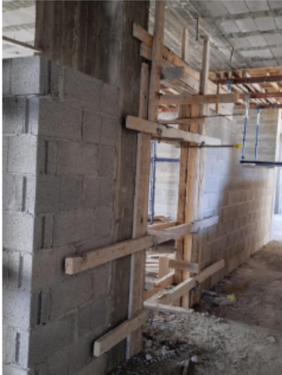
Formwork for door jambs and lintels
