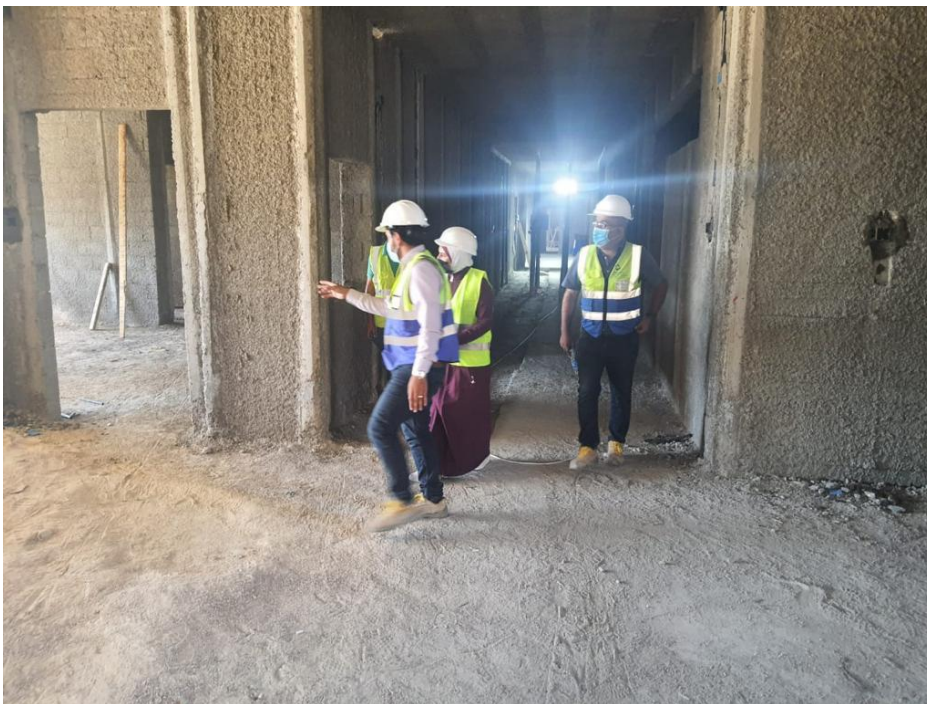
Eng. Ala'a/Medanat Site Engineer gave a brief about project components
