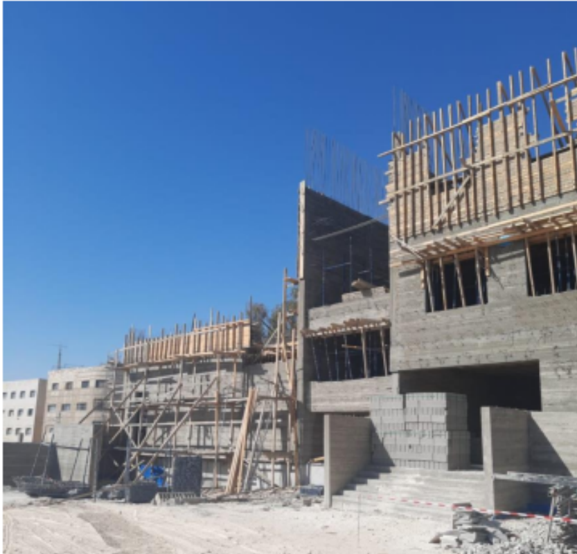
Formwork for external walls behind stone
