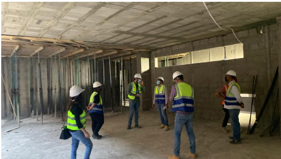
Checking work quality
