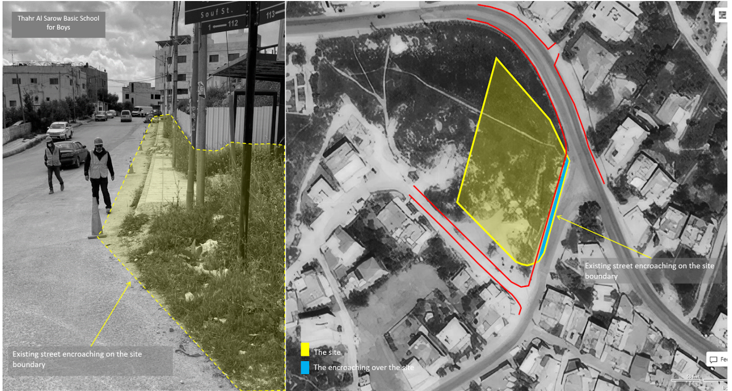
Figure 3. Existing street encroaching on the site boundary
