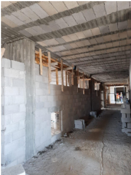
Formwork for lintels of internal windows
