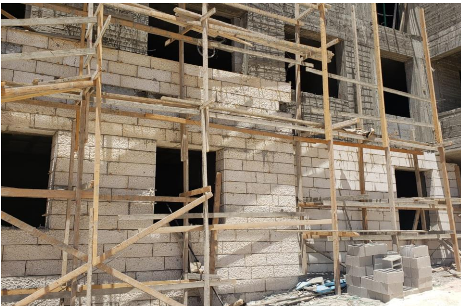
Removed defected stones
