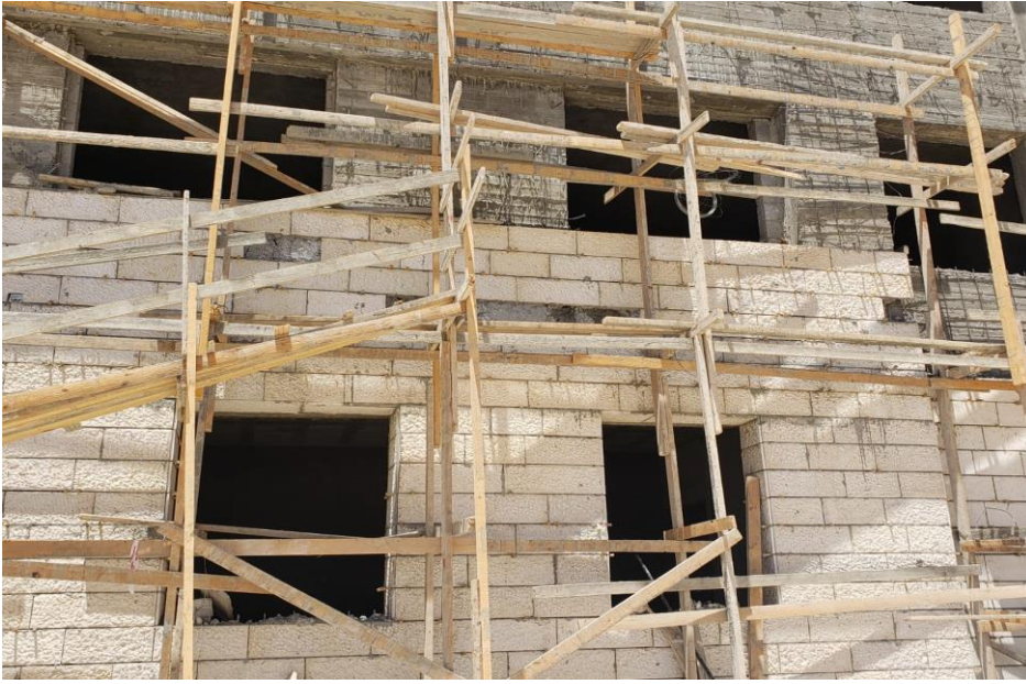
Removed defected stones
