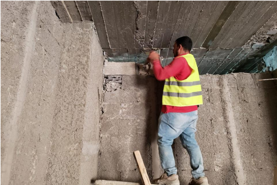
Replacing defected blockwork
