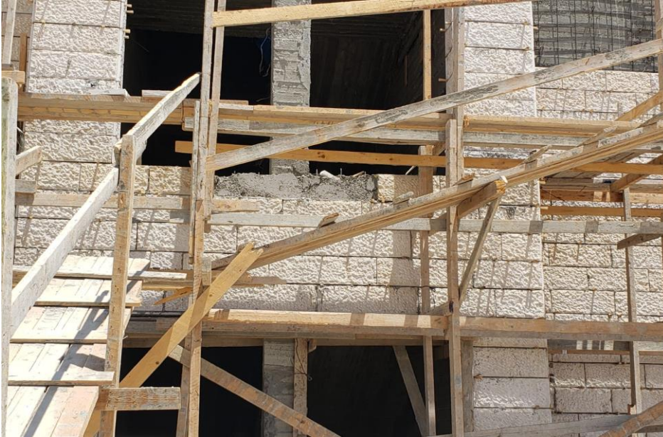
Removed defected stones
