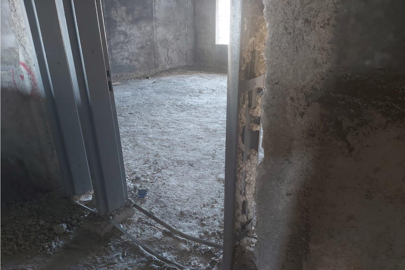
Starting to remove the defected door frame
