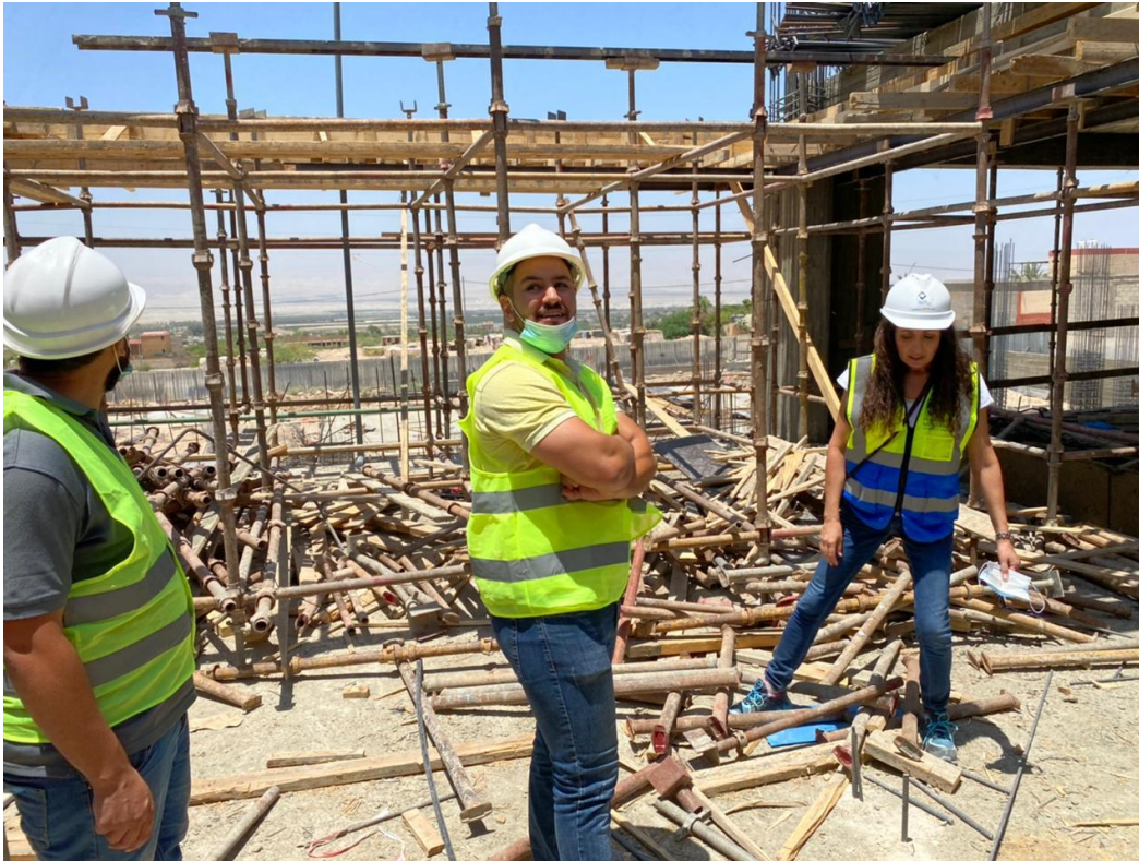
Slab formwork fixing for second floor zone (B)
