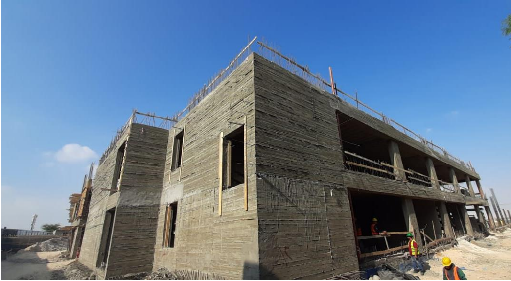
The quality of concrete works complies with specifications
