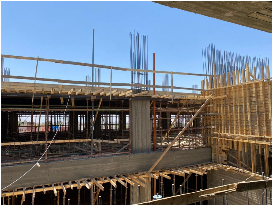
Preparation for casting of second floor slab zone (B)
