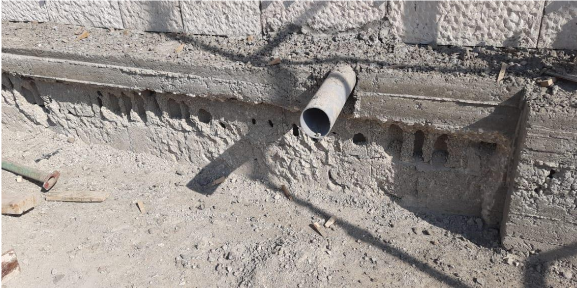
process to re-excute the expansion joint
