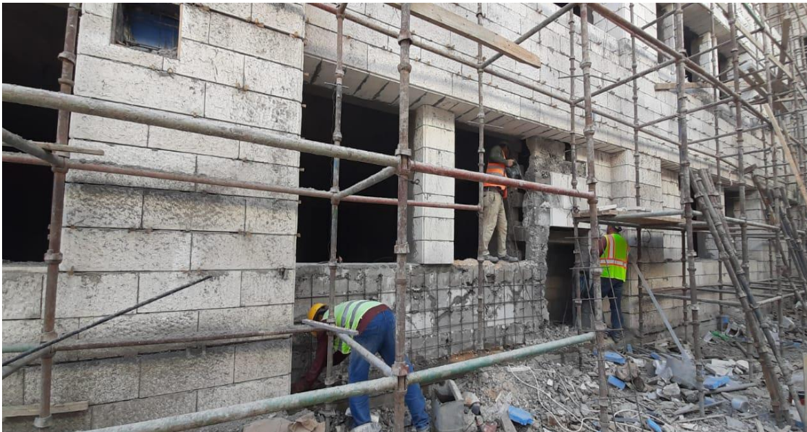
Finalizing the rectification for the elevation limit
