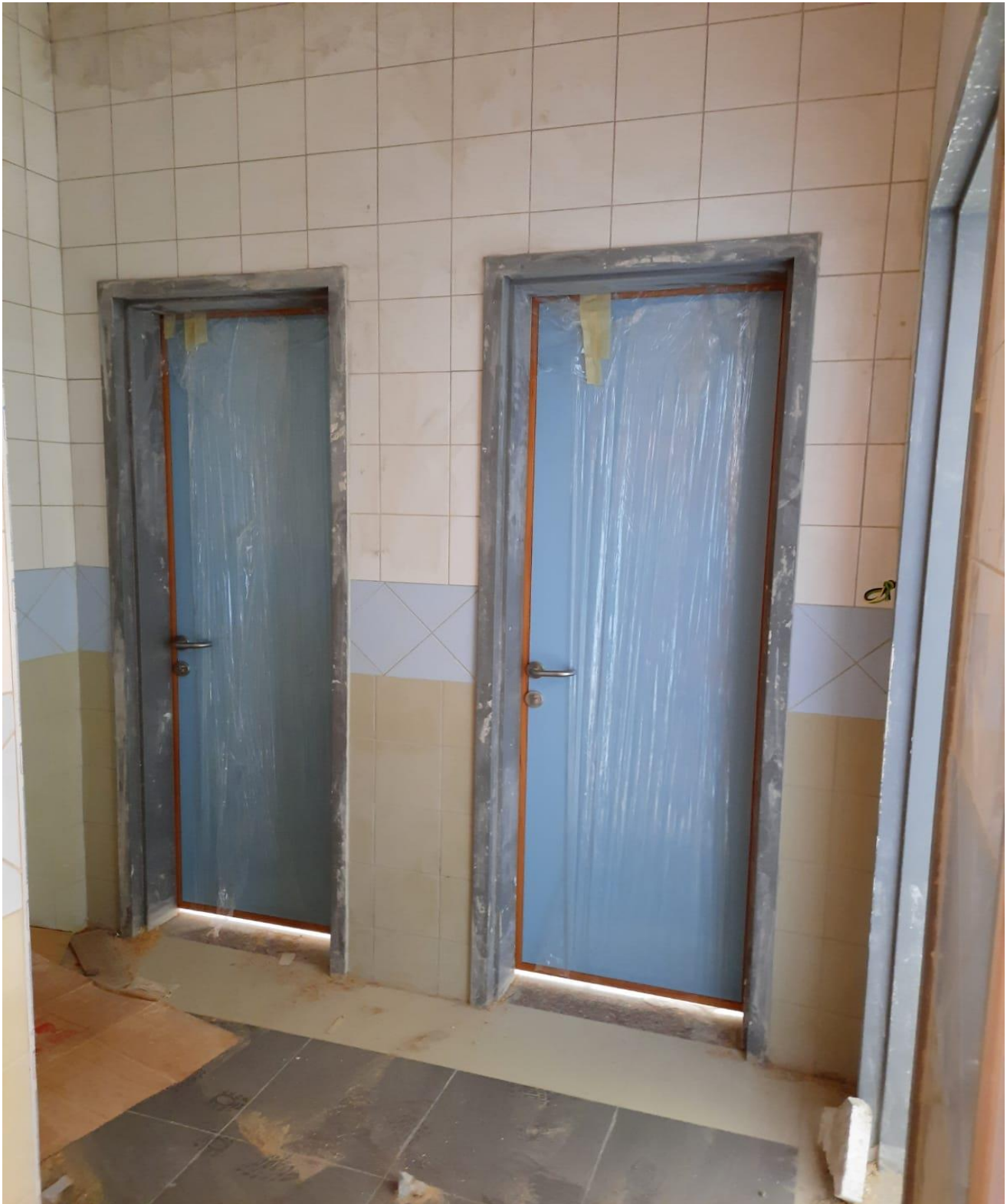
Re-tiling at the toilet
