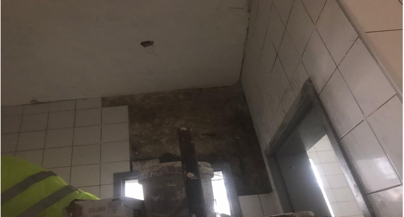
Removal of defected tiles
