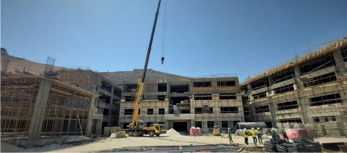
General view of the casted slab of the roof floor
