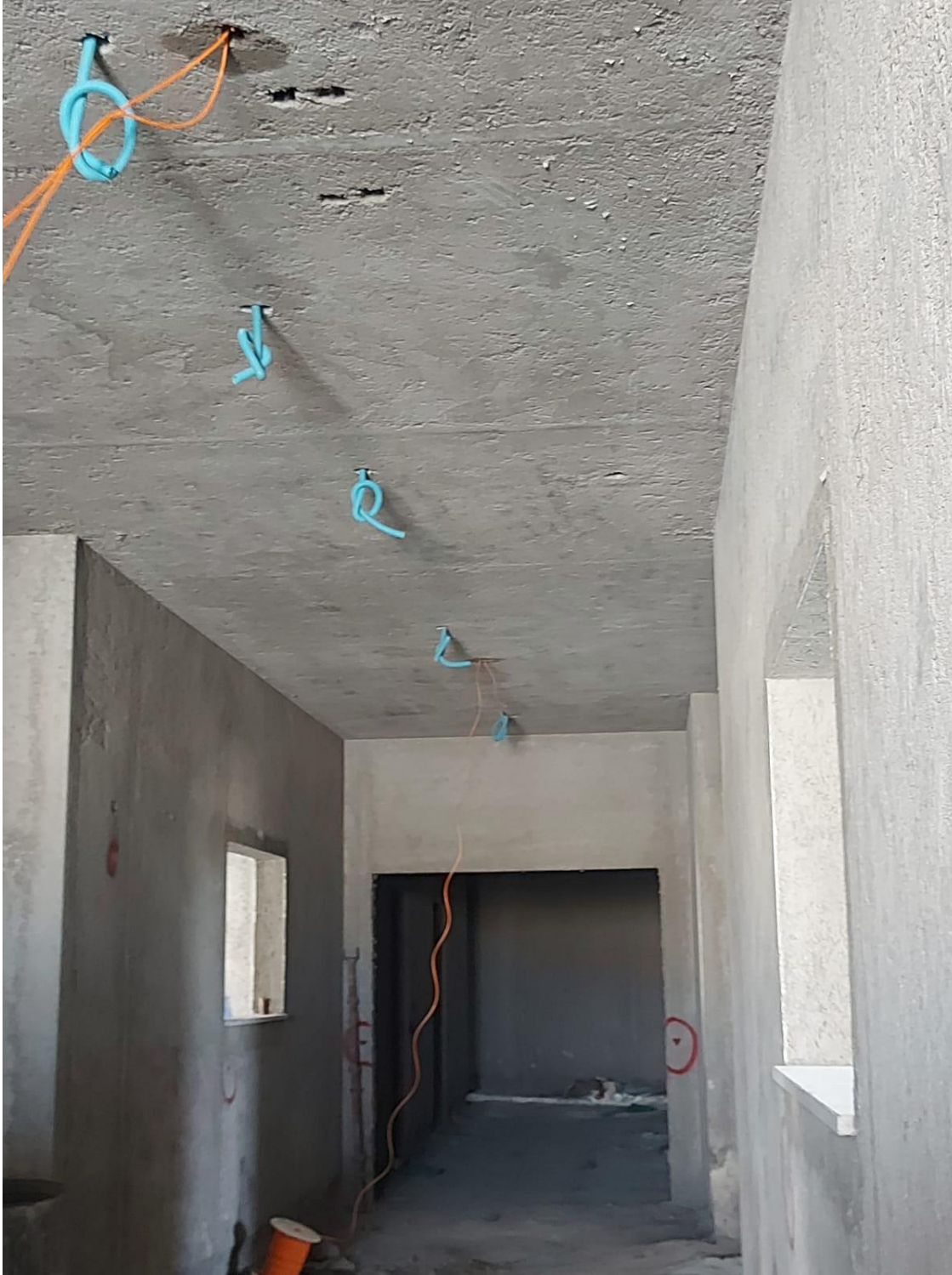
Starting electrical first fix for ground floor Zone "A"
