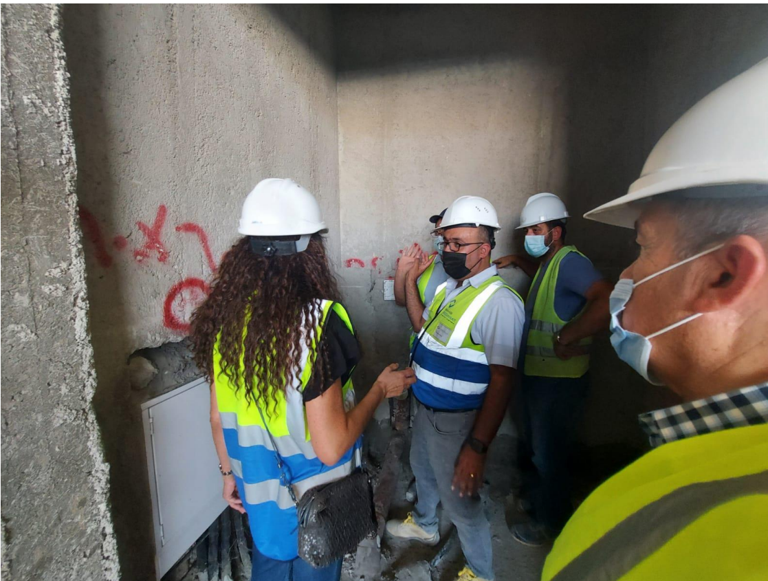
Discussing the appropriate way to install walls tiles
