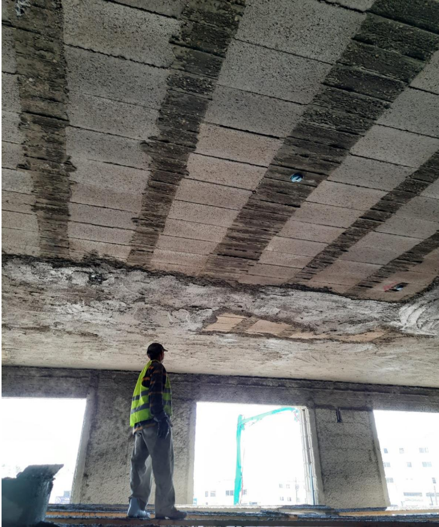
Executing second plastering layer before the first plastering layer
