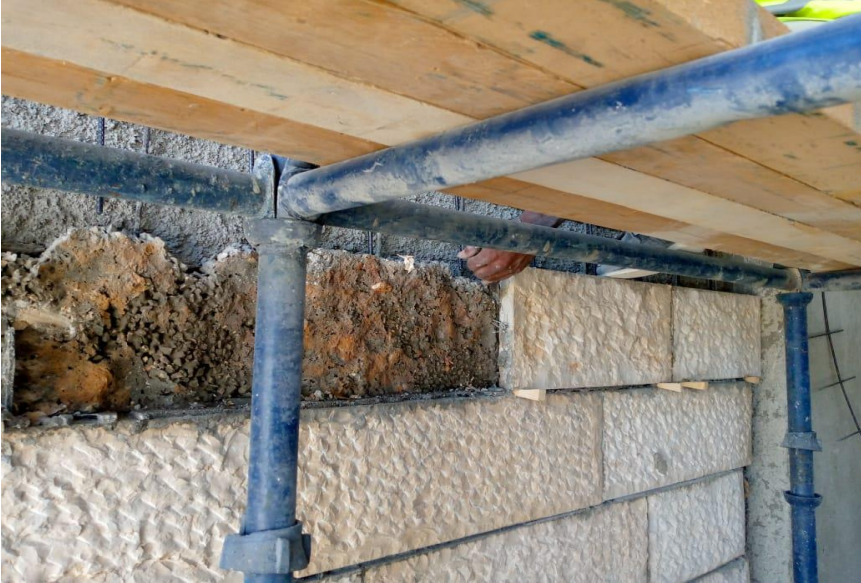
Removal of non-complying stone
