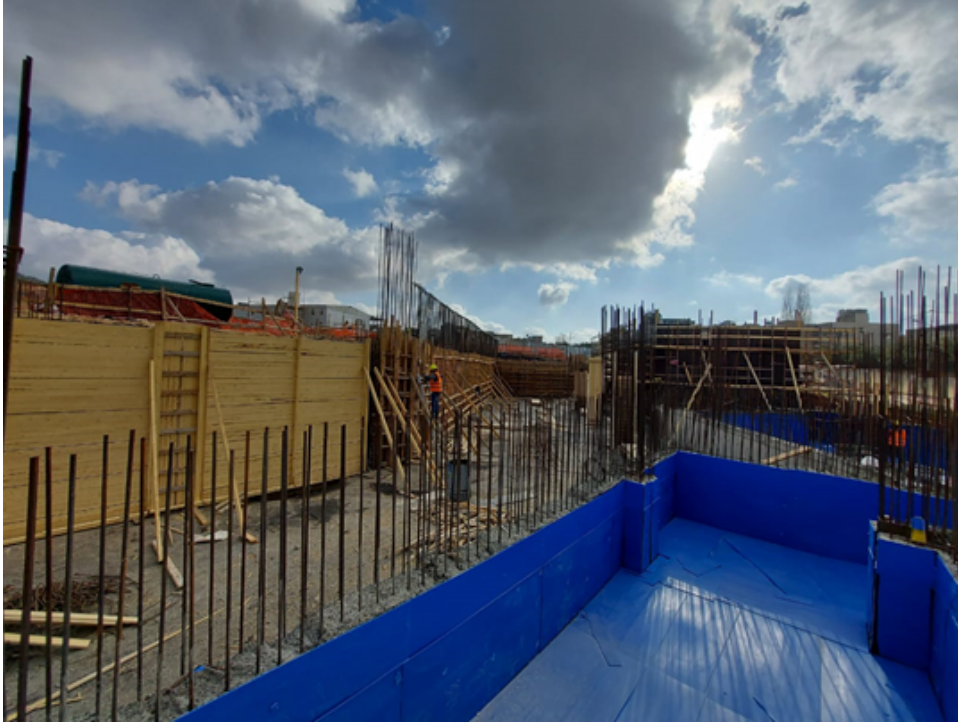
Cartonal fixation and basement wall formwork
