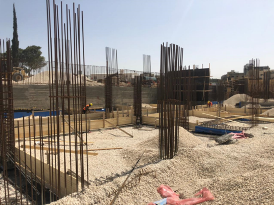
Ground beam formwork
