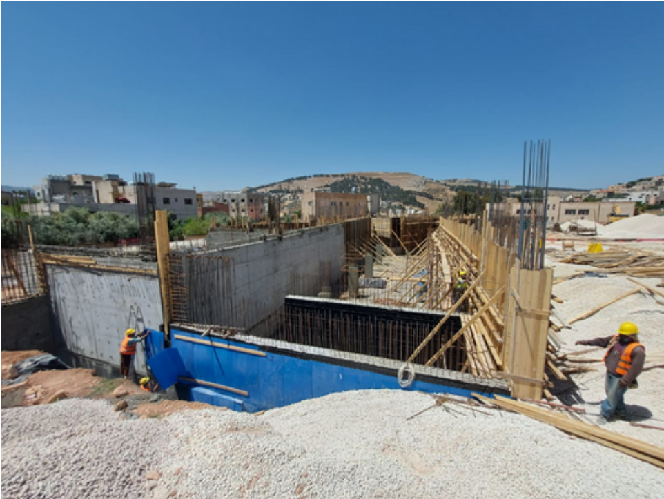
General View of the Project site
