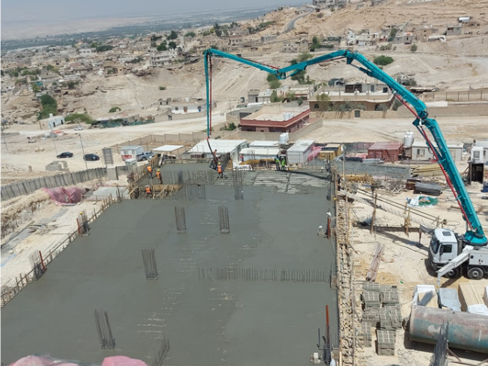
Casting of concrete for first floor slab
