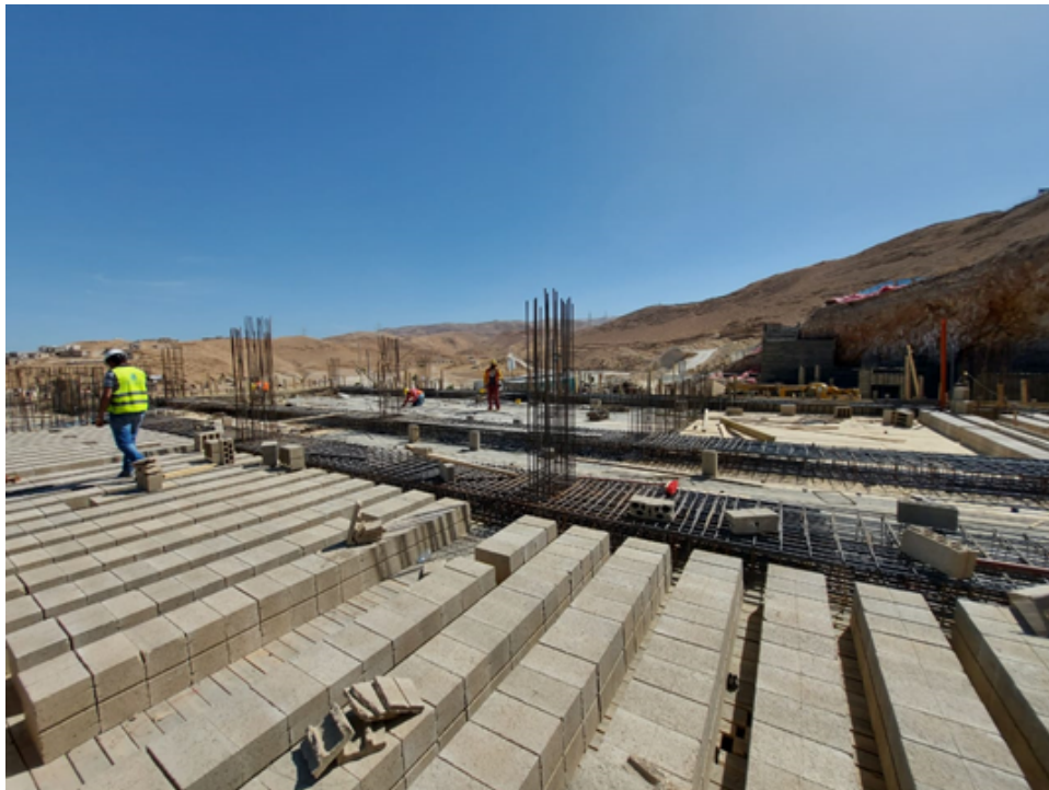
Formworks and steel reinforcement for slab of school building zone (A)
