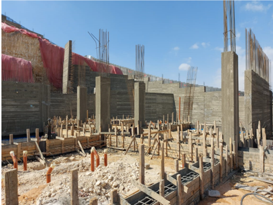
School building zone (A) tie beams and mechanical works
