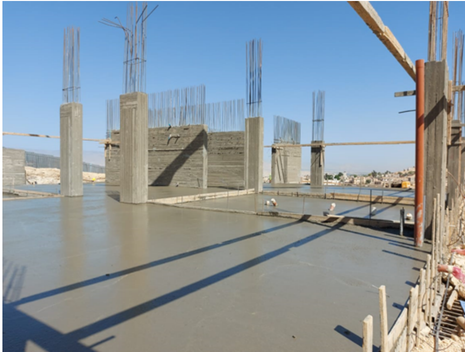
Concrete Casting for school building zone (A) Slab on grade
