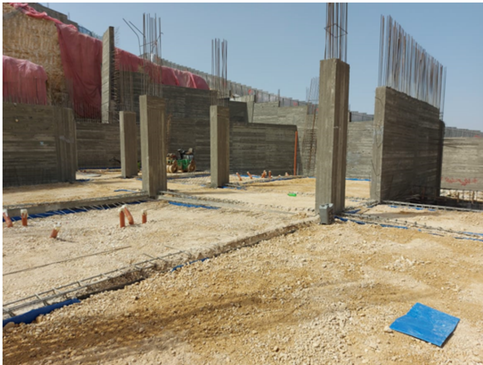
Backfilling works for school building zone (A)
