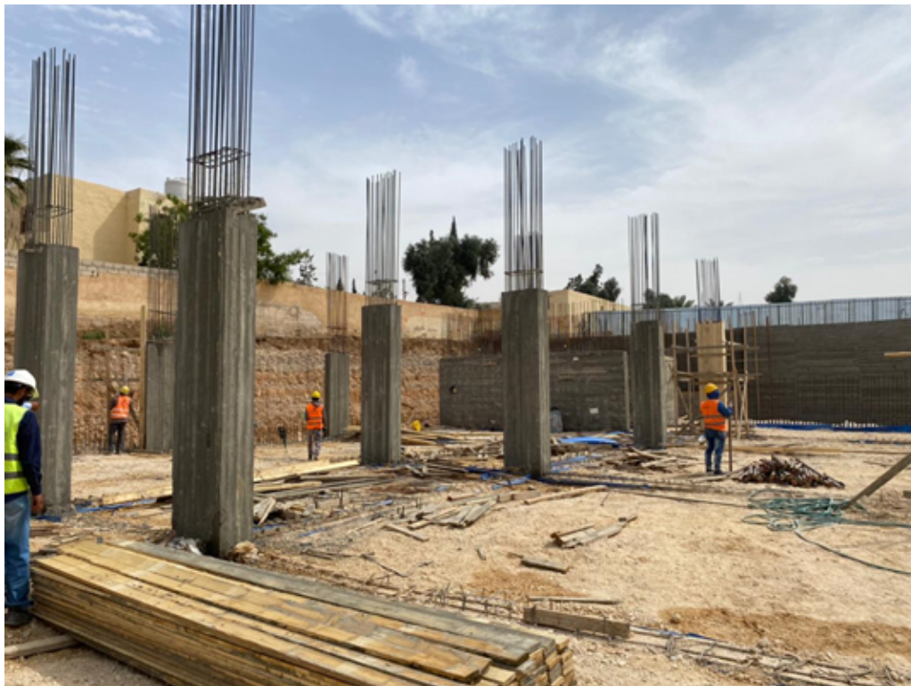
De-shuttering for ground floor columns
