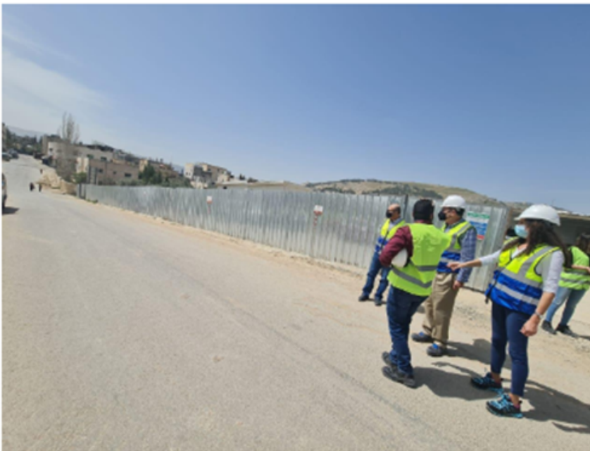
There is an encroaching of neighbor wall towards the school boundary plot.
