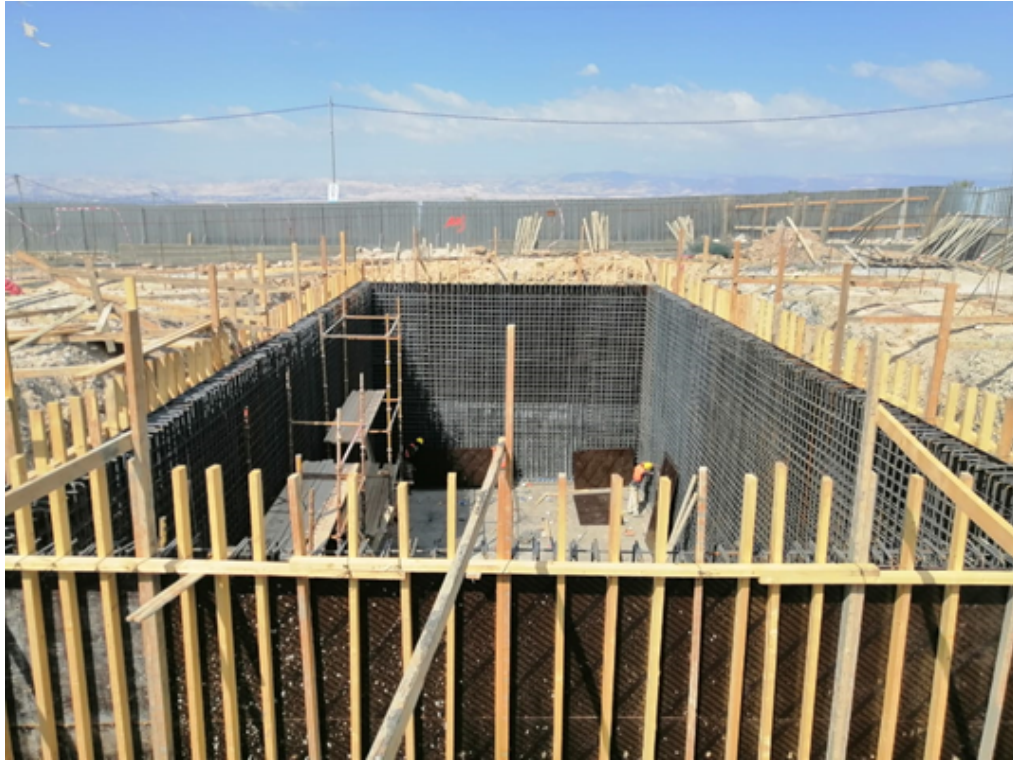
Sewage collection formwork and steel reinforcement
