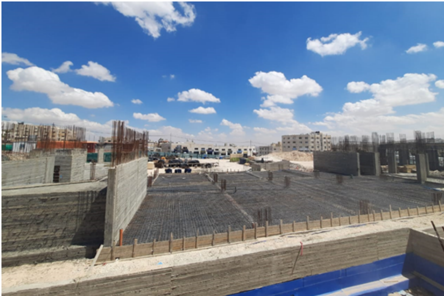
Steel reinforcement for Slab on grade
