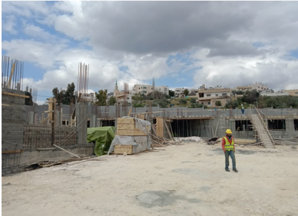
Ground floor slab formwork Part (1)
