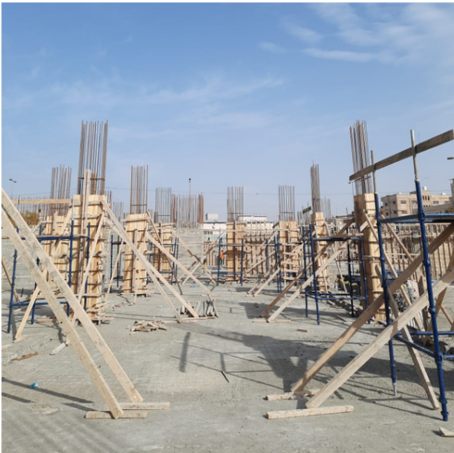
Ground floor columns' formwork
