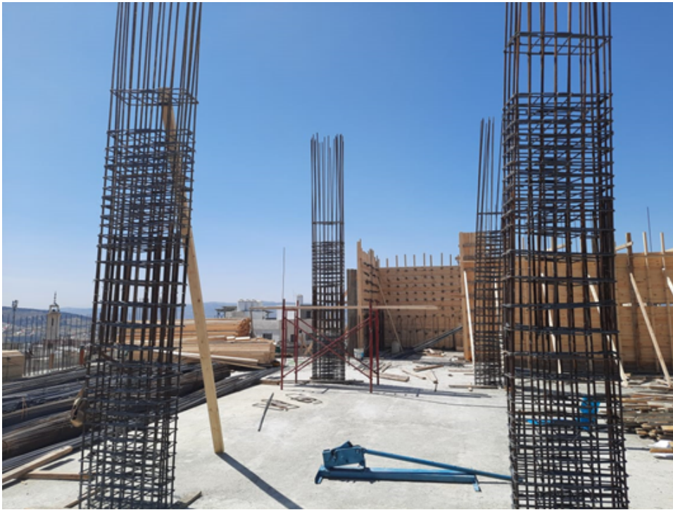
Steel reinforcement for second floor columns
