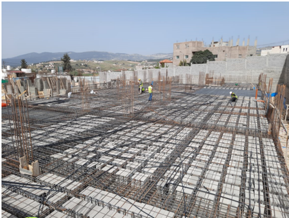
Ground floor slab steel reinforceme nt and electrical work part (1)
