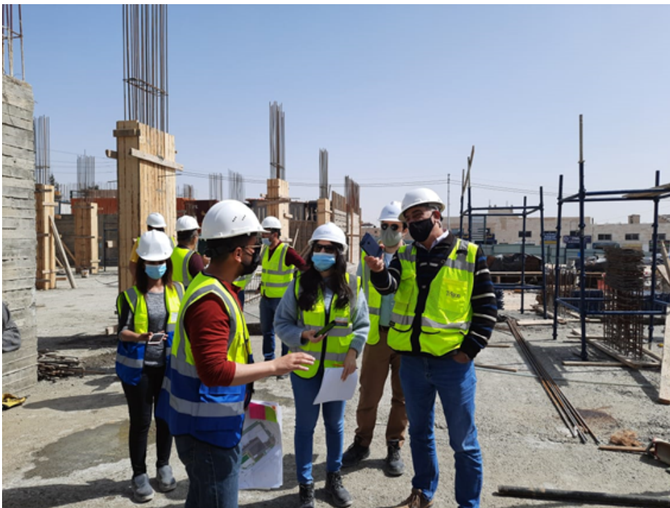
Discussing work progress and Quality check of executed works
