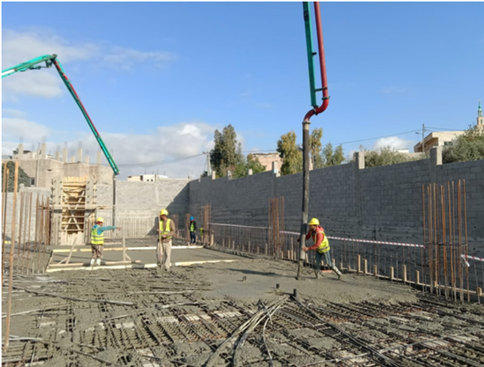
Casting concrete for ground floor slab part (1)
