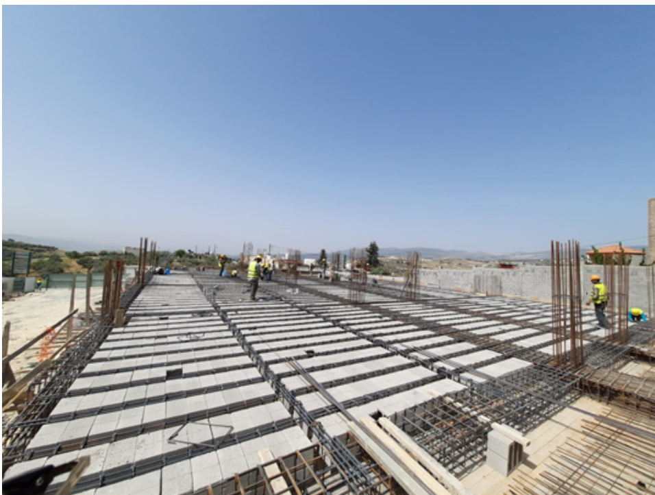
Steel reinforcement for ground floor slab part (2)
