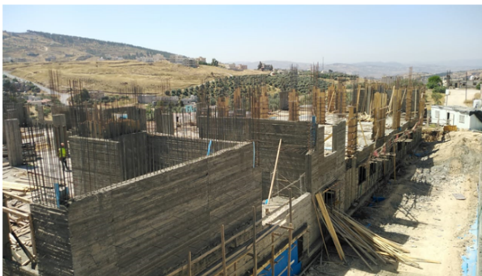
General View of Project site
