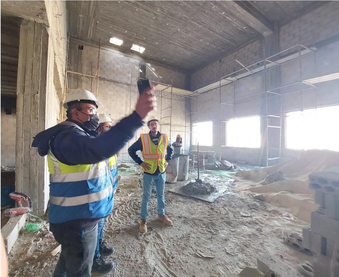
The team inspected the blockwork going on in the multi-purpose hall
