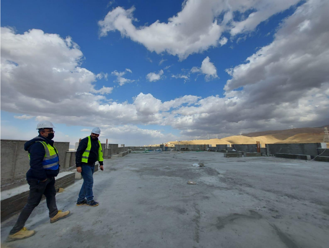
The team inspected the preparation work for insulation at the roof
