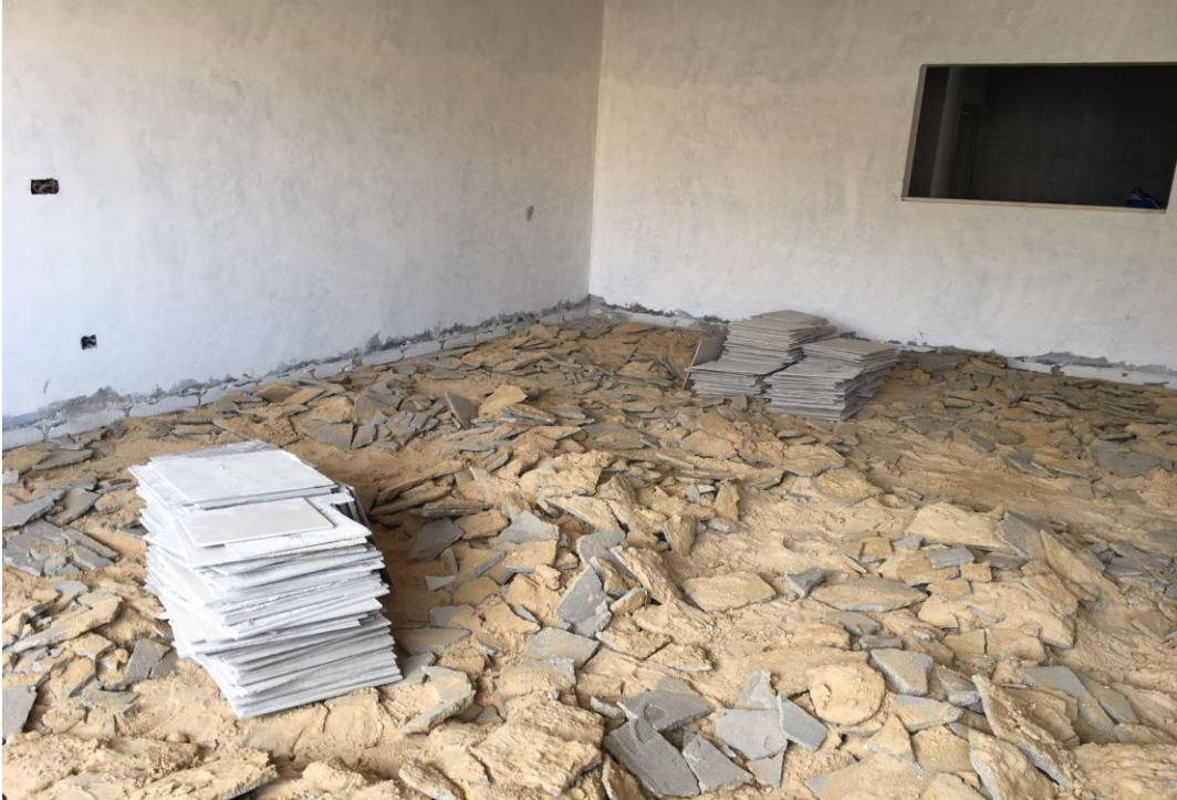
Starting with the demolition of porcelain floor tiles
