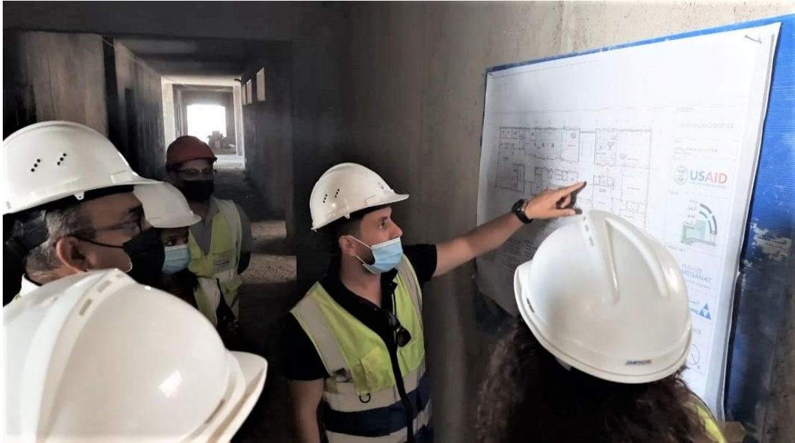
The Consultant's site engineer gave a brief about the ongoing activities
