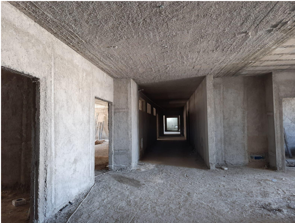
General view showing the plastering work
