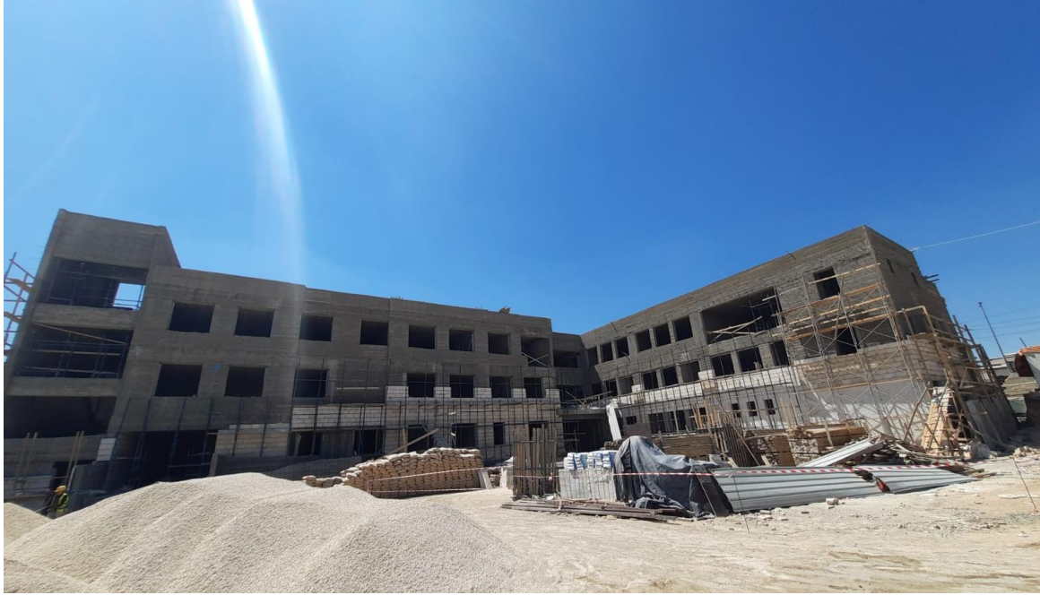
General view of the completed roof floor casting (the last slab)
