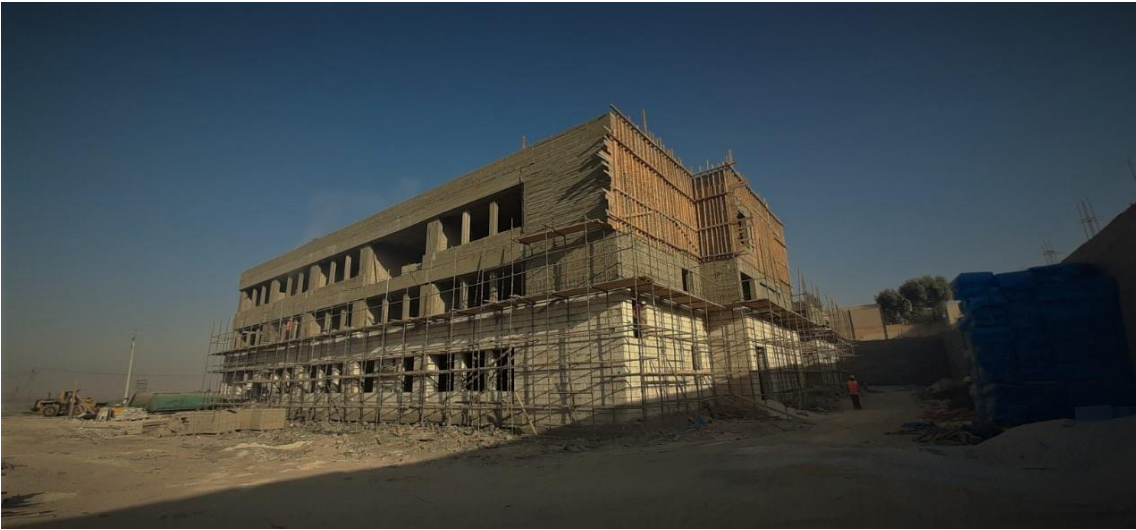
General view of the project
